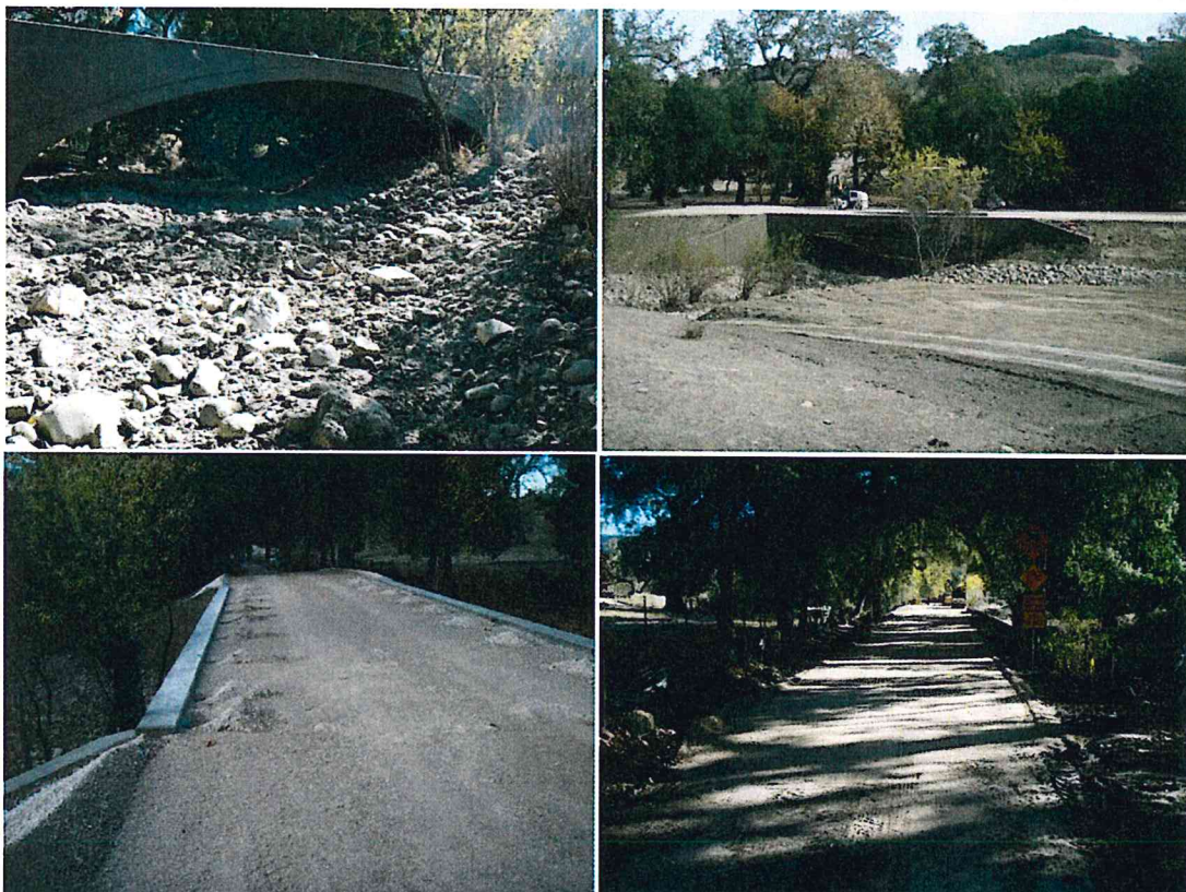
Figure 7: Backfilling the arches and soil anchors.
