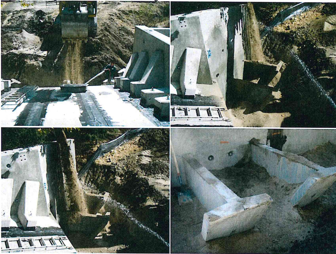
Figure 7: Backfilling the arches and soil anchors.
