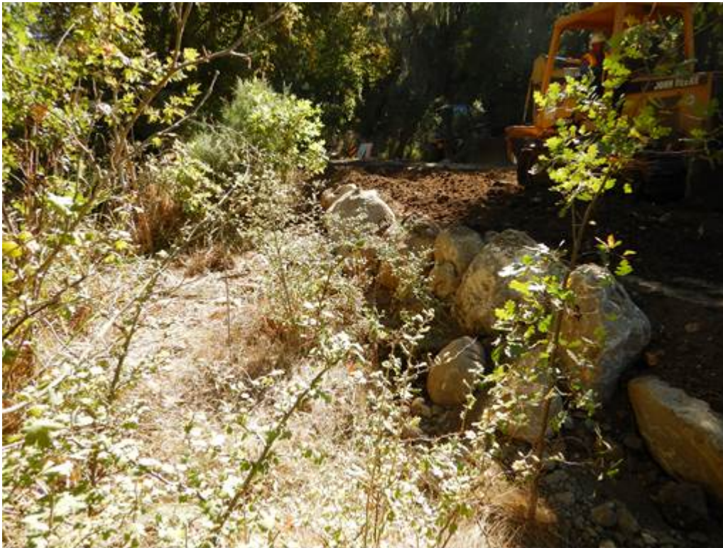
Figure 4: Rock tree wells installed to hold up the road embankments.
