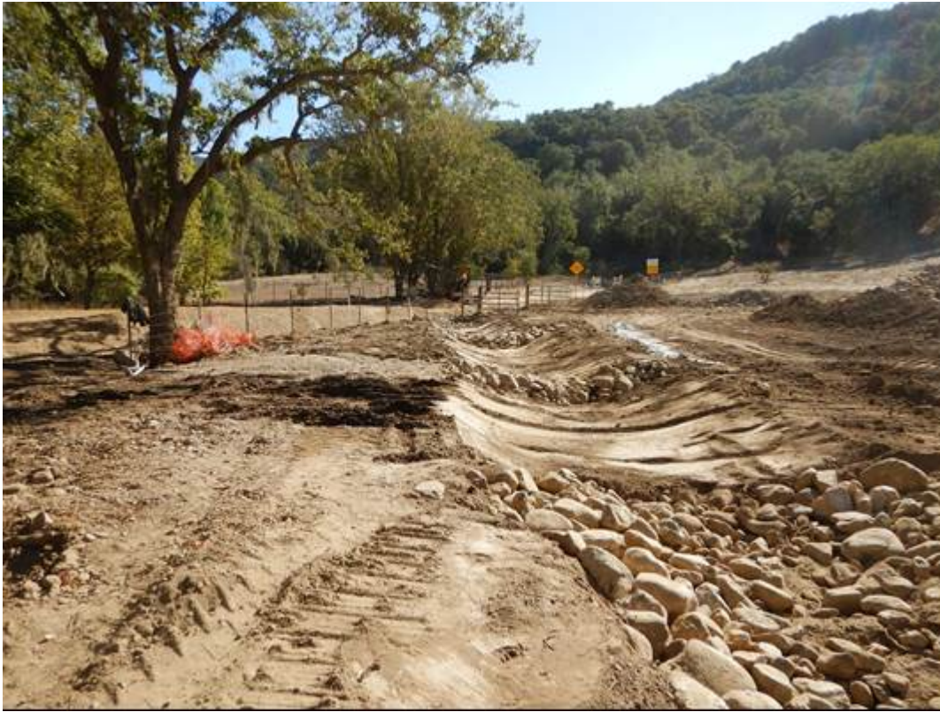
Figure 9: Road drainage swale on the south side of the bridge.
