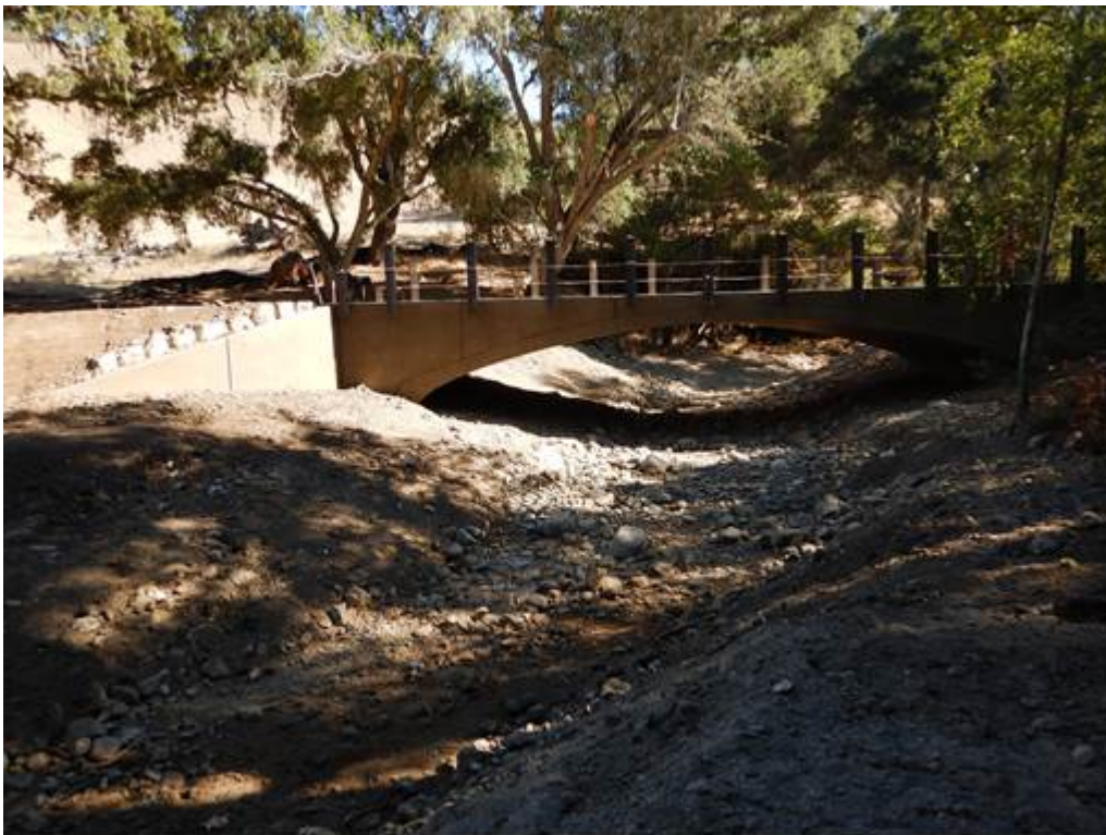
Figure 2: Bridge staining and graffiti proofing with installed bridge rain posts.
