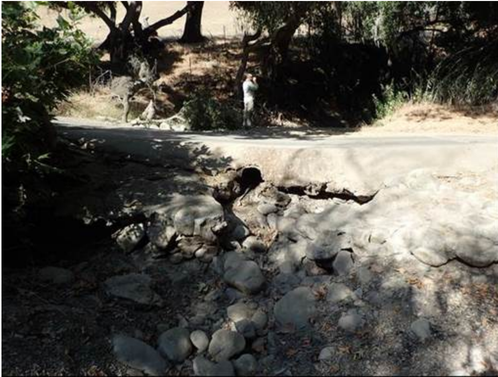
Figure 1: Pre-project condition looking upstream.
