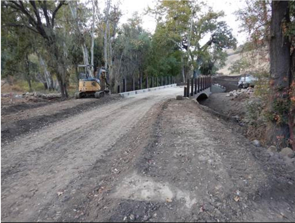
Figure 3: Installed 4 foot wide shoulders where the guardrails will be placed.
