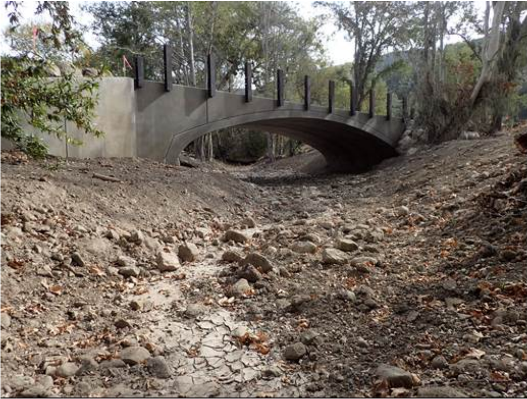
Figure 7: Stained and anti-graffiti proofed bridge with installed bridge rail posts.
