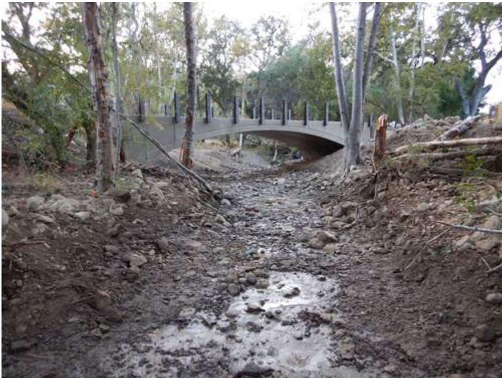
Figure 2: Completed stream work.
