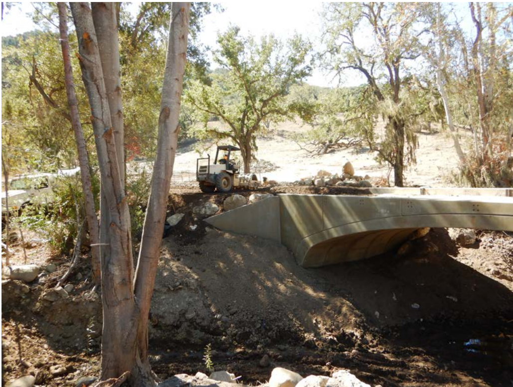
Figure 4: Working on widening the road shoulders to 4 feet.
