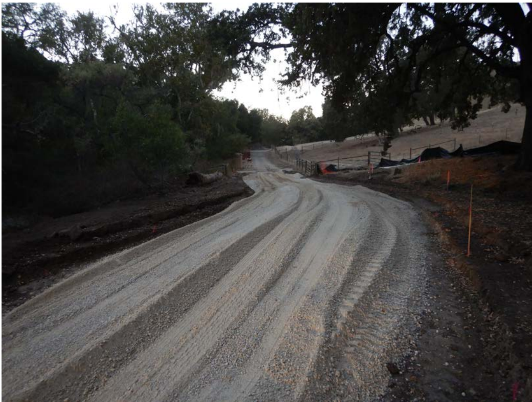
Figure 6: Laying out the road-base.
