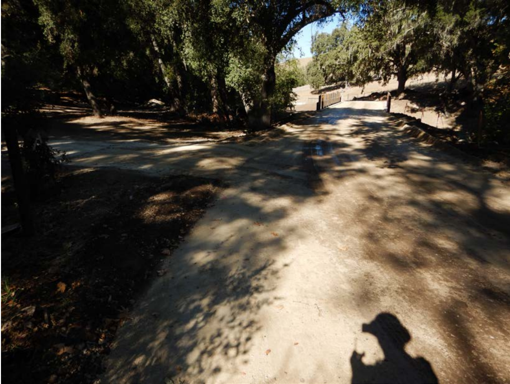
Figure 7: Completed installation of the road-base and ready for paving.
