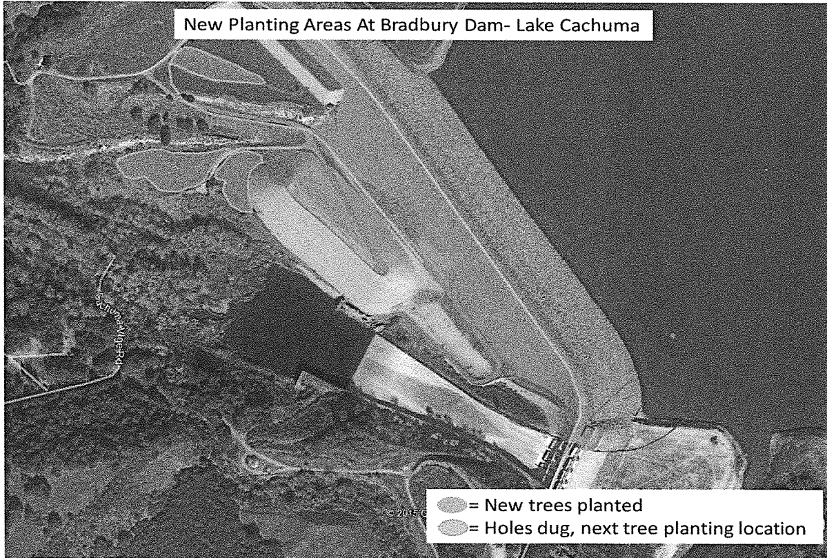
Exhibit C: Aerial view of designated planting locations at Bradbury Dam, Lake Cachuma.
