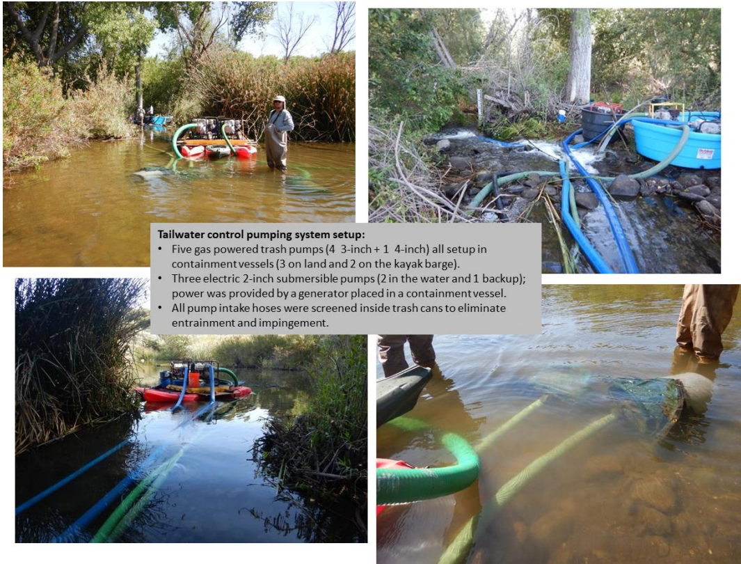
Figure 3: Setup and operation of the pumping system.
