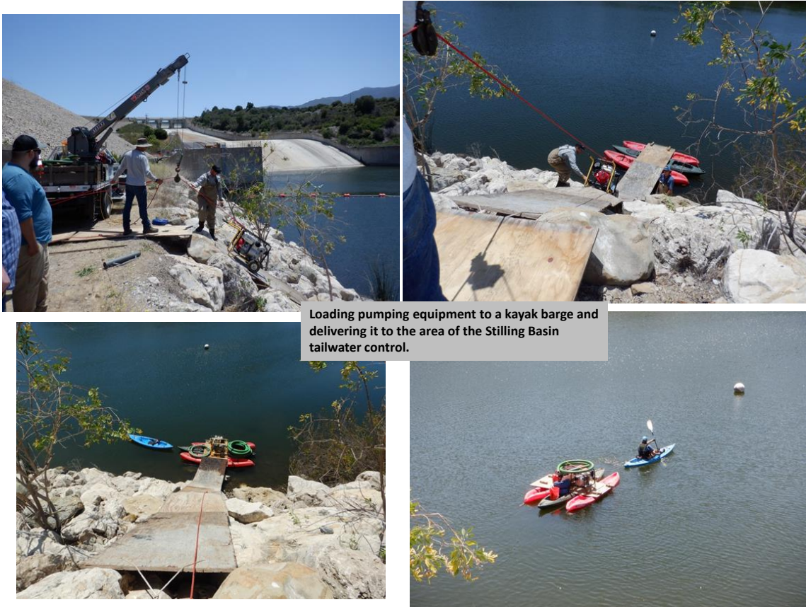
Figure 2: Delivery of the pumping system to the Stilling Basin tailwater control.
