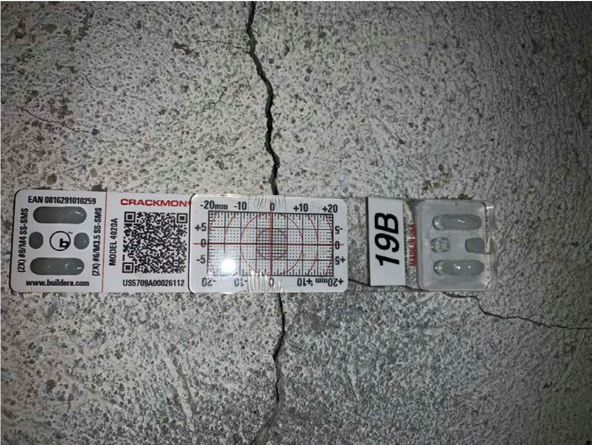
Crack Monitors installed on Lauro Outlet Works Anchor Piers
