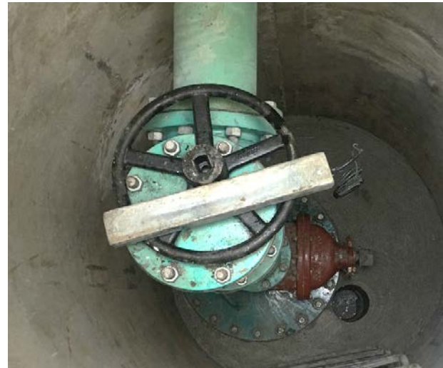
Blowoff 504+65 After (anode to be installed)
