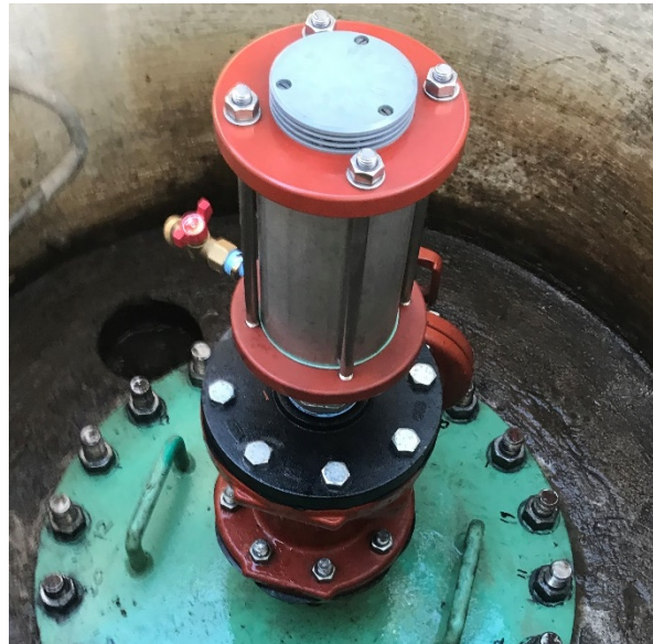
Access Hole 295+50 After (with 4" outlet for sampling and injection)
