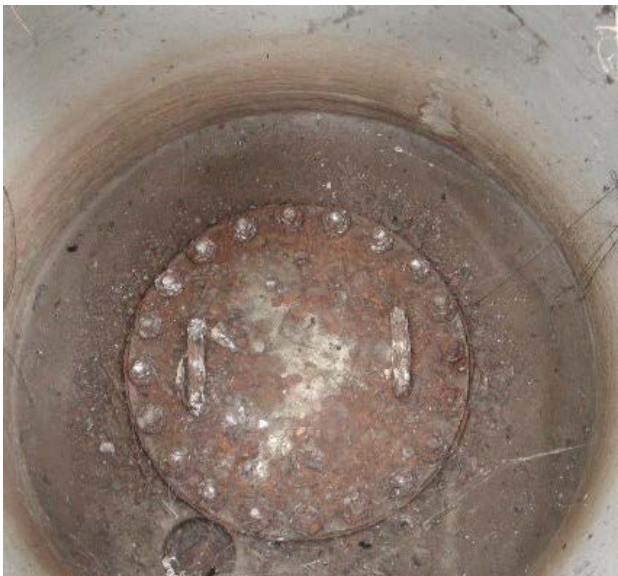
Access Hole 295+50 Before
