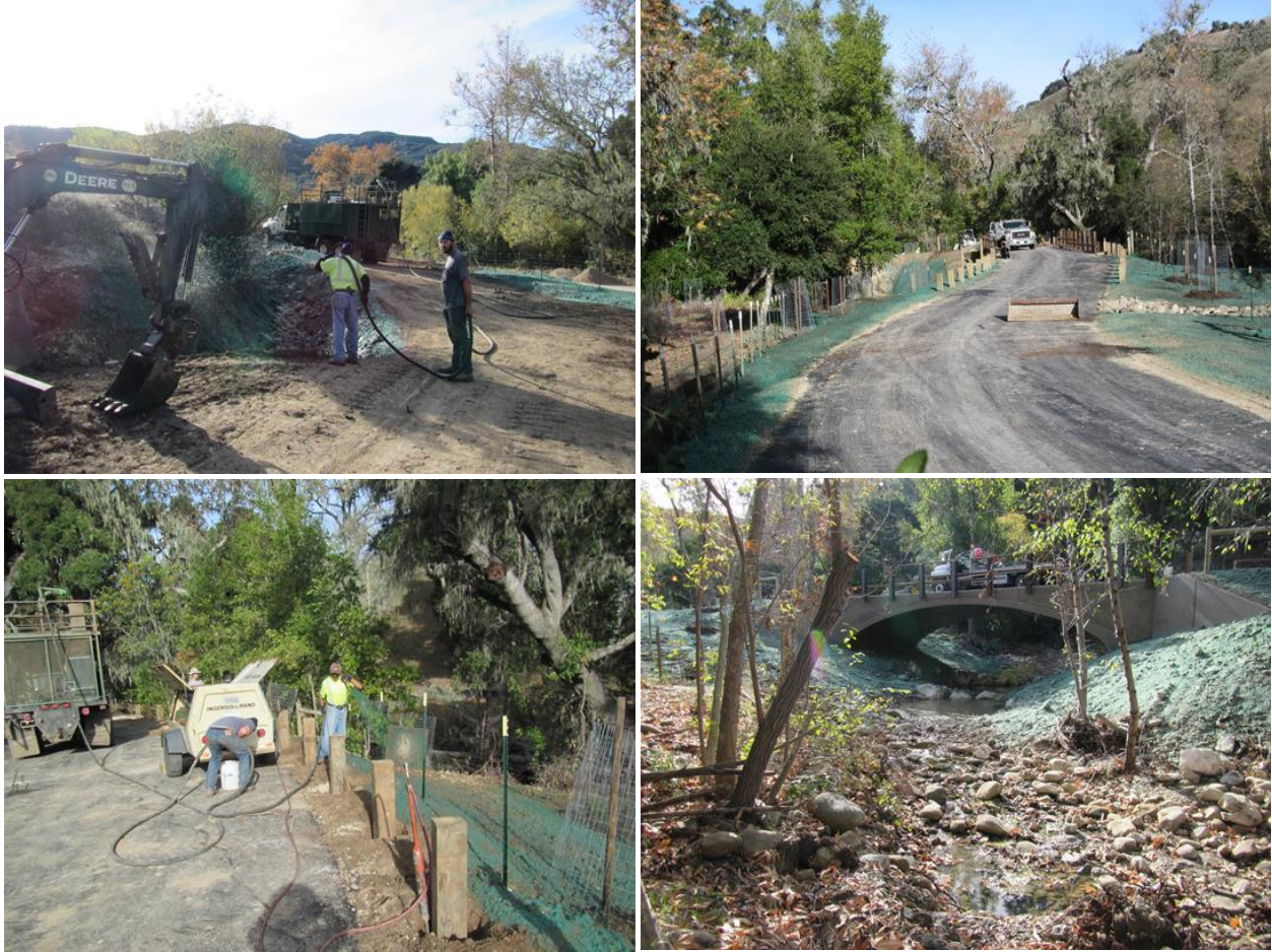
Figure 4: Hydro-mulching/seeding of the site.
