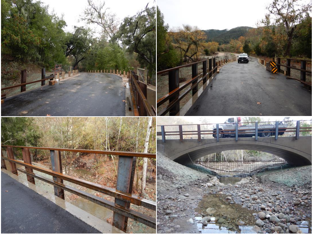
Figure 5: Guardrail and bridge rail work.
