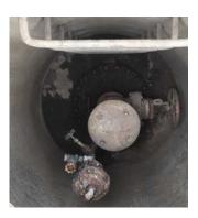
Corroded air-vac at Station 676+67
