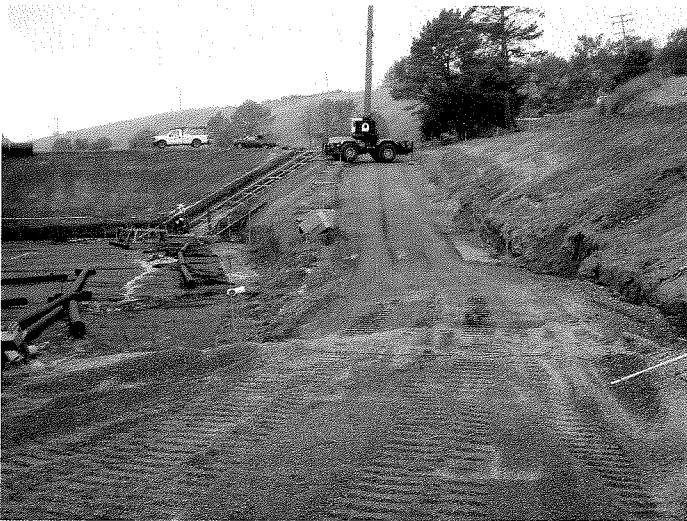
Picture 4 – Access Improvement progress
