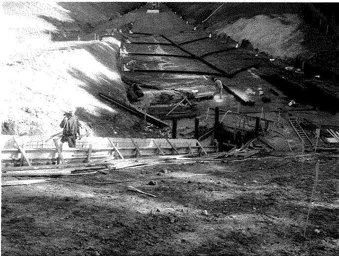
Picture 3 – Subdrain installation
