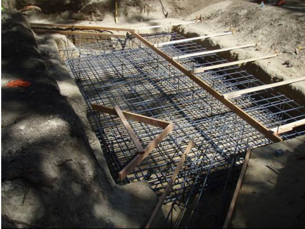
Figure 4: Foundation rebar placement.
