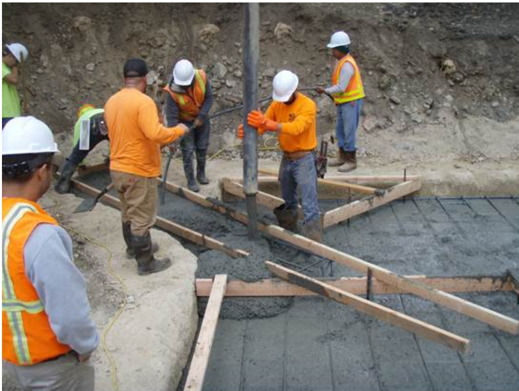
Figure 5: Pouring the foundations.
