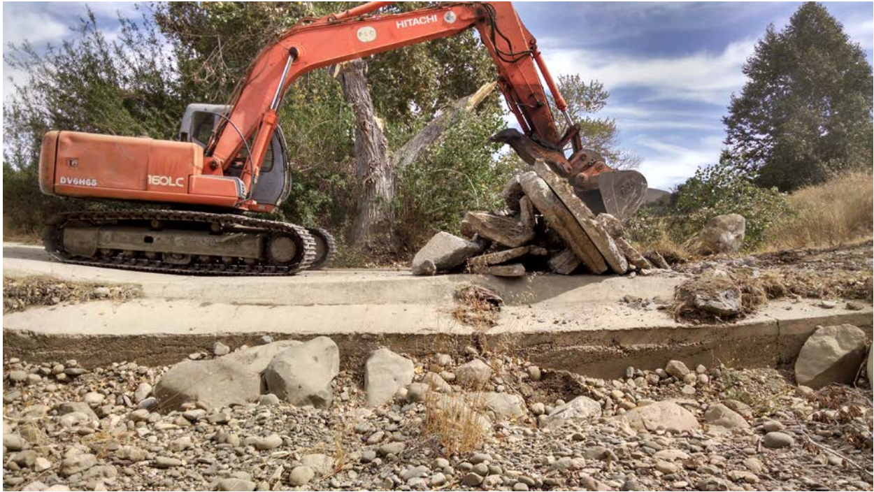
Figure 2: Removal of the concrete low flow crossing along S. Refugio Road.
