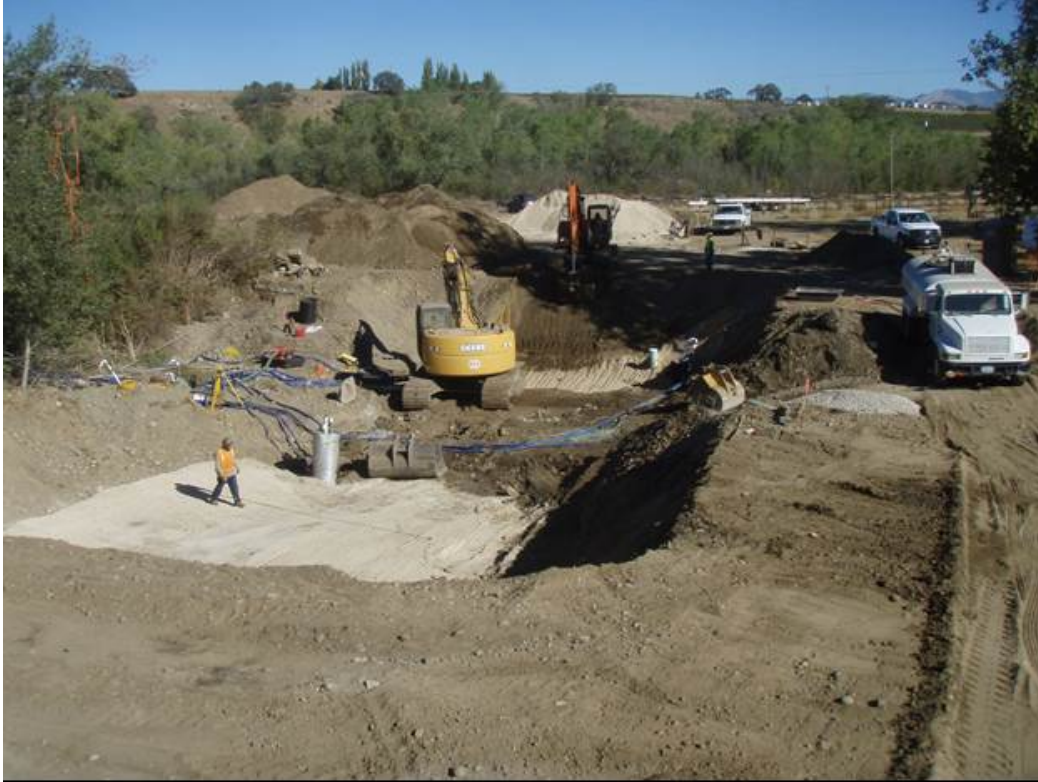
Figure 4: Preparing the sub-foundation for forming the foundations.
