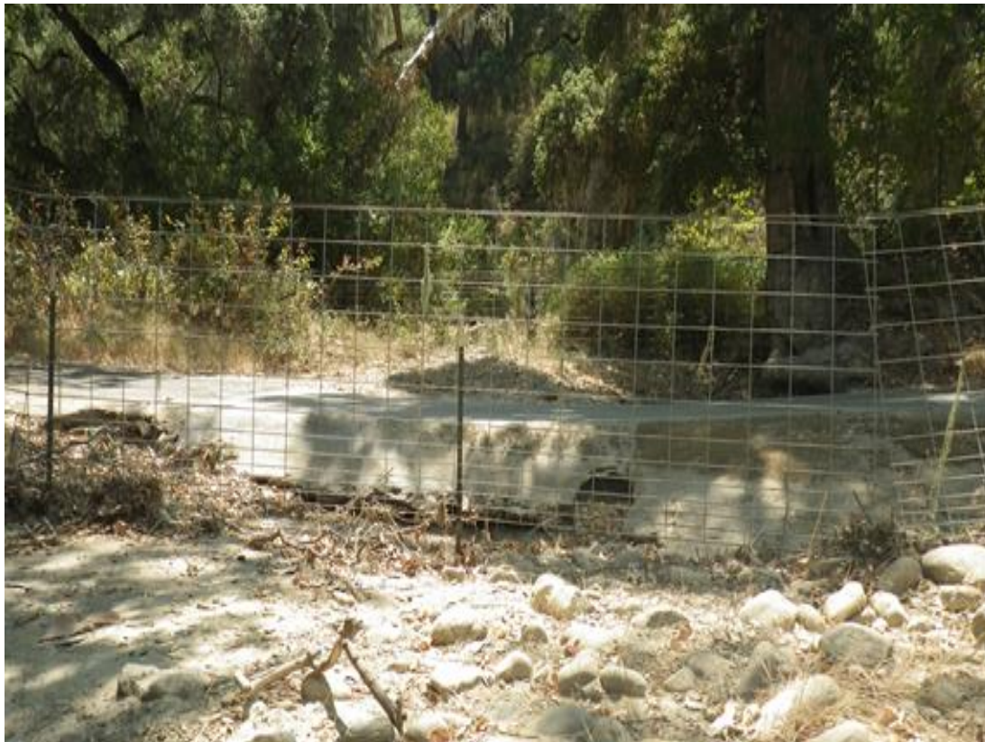
Figure 1: Pre-project condition looking upstream.
