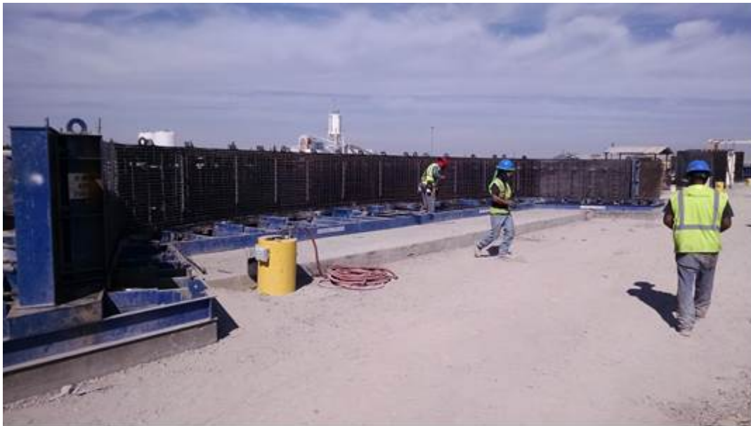
Figure 7: Arch construction at Bethlehem.
