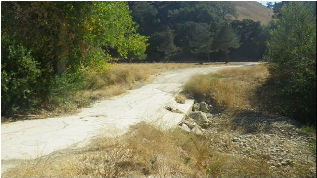
Figure 1: Pre-project condition looking upstream.
