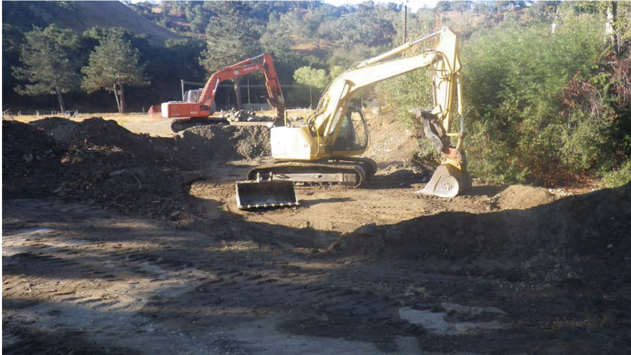
Figure 3: Excavations for the bridge foundations.
