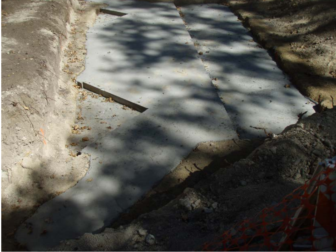
Figure 6: Completed foundations.
