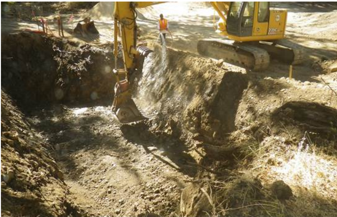
Figure 3: Excavations for the bridge foundations.
