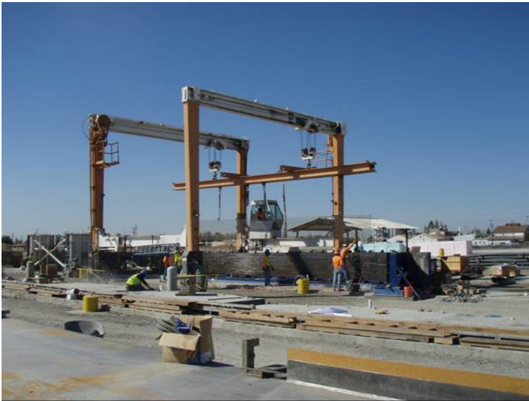
Figure 5: Arch construction at Bethlehem.
