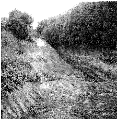
Picture 1 –Lauro Retention Basin Overview Pre-Construction
