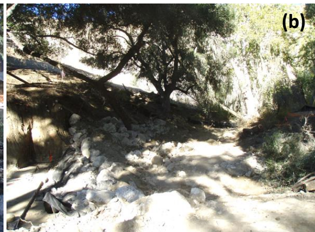
Figure 8: Change Order 1 work as directed by onsite HDR engineers; (a) moving the willow tree to the right bank and (b) installing the bank slope protection just upstream of the bridge foundation.
