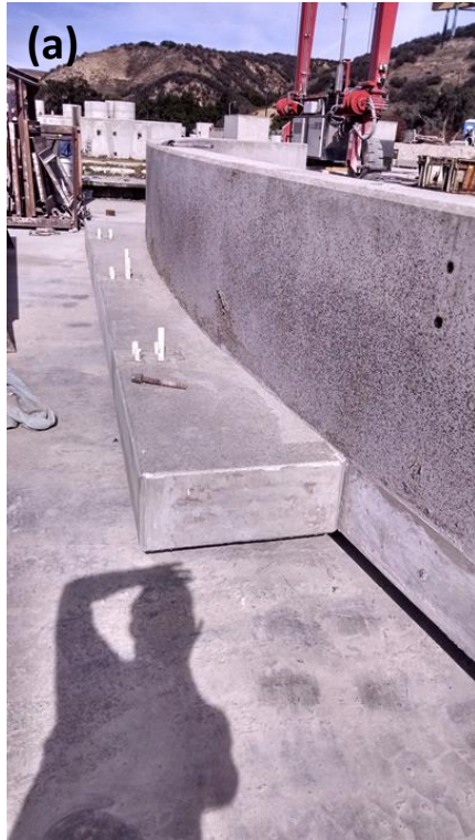
Figure 5: Pre-Con bridge fabrication of (a) completed arch with headwall and (b) delivery of that arch over the Santa Ynez River in route to the project site on 10/29/15.
