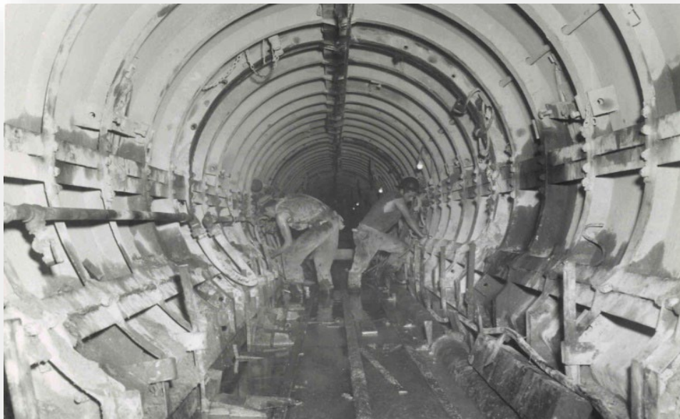
Tecolote Tunnel Construction
