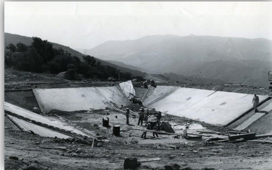
Construction of Bradbury Dam
