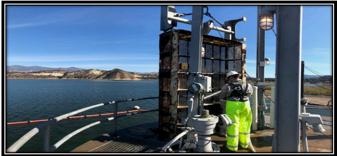
North Portal Intake Tower
