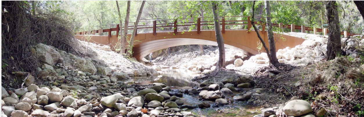
Quiota Creek Fish Passage Project
