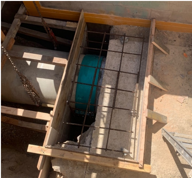
External repair clamp reinstalled and reinforced
