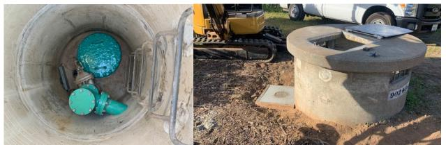
**Figure 3.** Blowoff Structure 902+96 – Left - piping replaced, nozzle and access lid coated and anodes installed. Original valve needs to be replaced in future shutdown. Right – Outside valve installed on the blowoff.
