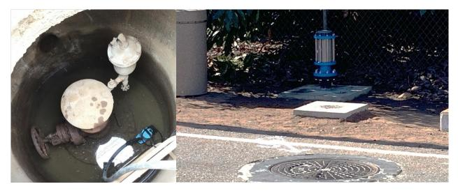
**Figure 3.** AVAR Structure 874+00 – Left – original subgrade AVAR valve with unknown function in Highway 192. Right - AVAR valve replaced and raised above grade.
