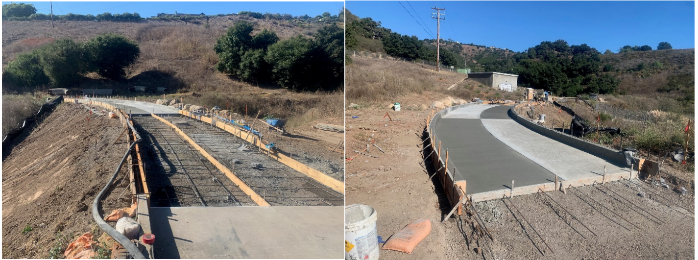
Figure 2. Lauro Reservoir Bypass Channel Road Repair - (a) washout and cantilevered concrete channel and manhole after 2023 storm event; (b) backfill and compaction of washout; (c) forms and rebar for replacement concrete channel; (d) concrete channel extension poured to mitigate for future damages.
