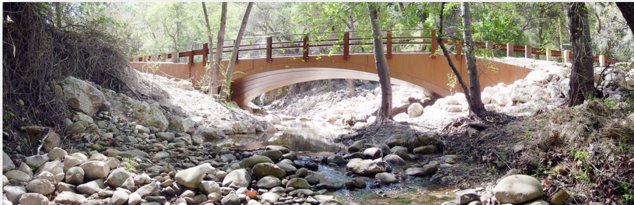
Quiota Creek Fish Passage Project
