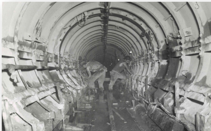
Tecolote Tunnel Construction
