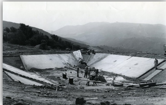
Construction of Bradbury Dam
