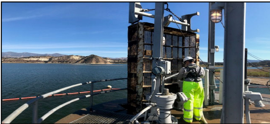
North Portal Intake Tower
