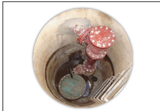
Figure - Inside of Blow Off Structure
