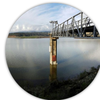
Figure - North Portal Intake Tower
