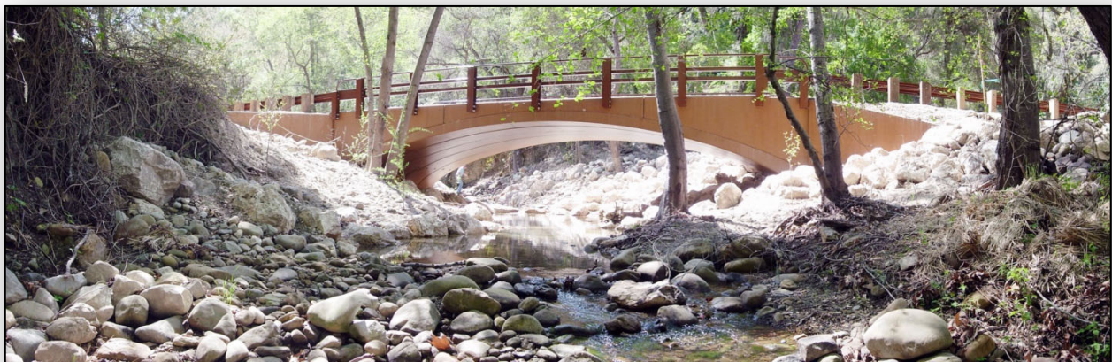
Quiota Creek Fish Passage Project
