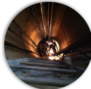
Figure - North Portal Elevator Shaft
