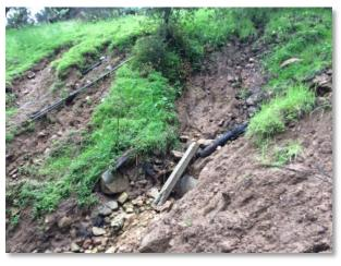
significant risk to system operation. This project would consist of securing the conduit at this location and restoring appropriate sediment over the pipeline on the slope in order to eliminate the risk associated with the continued hillside erosion during storm events. The location of the exposed pipeline, SCC, Right-of-Way, and existing access route is shown in the Exhibit 1.
