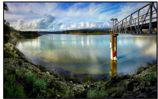
Tecolote Tunnel Intake Tower, Lake Cachuma
