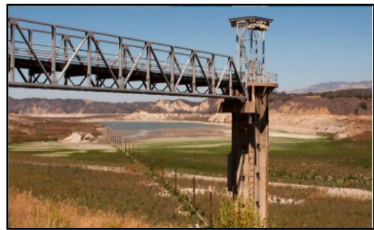
Tecolote Tunnel Intake Tower, Lake Cachuma
