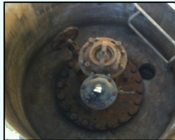
Air Vent 352+07 Before
