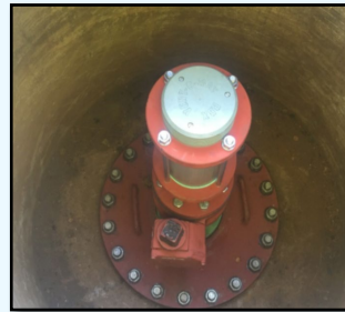
Air Vent 352+07 After
