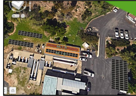
COMB Office Building
