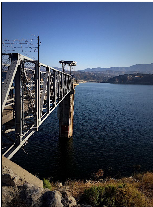
Tecolote Tunnel Intake Tower, Lake Cachuma
