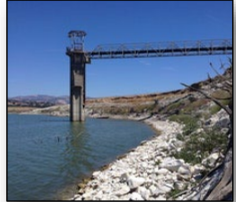
Tecolote Tunnel Intake Tower, Lake Cachuma
