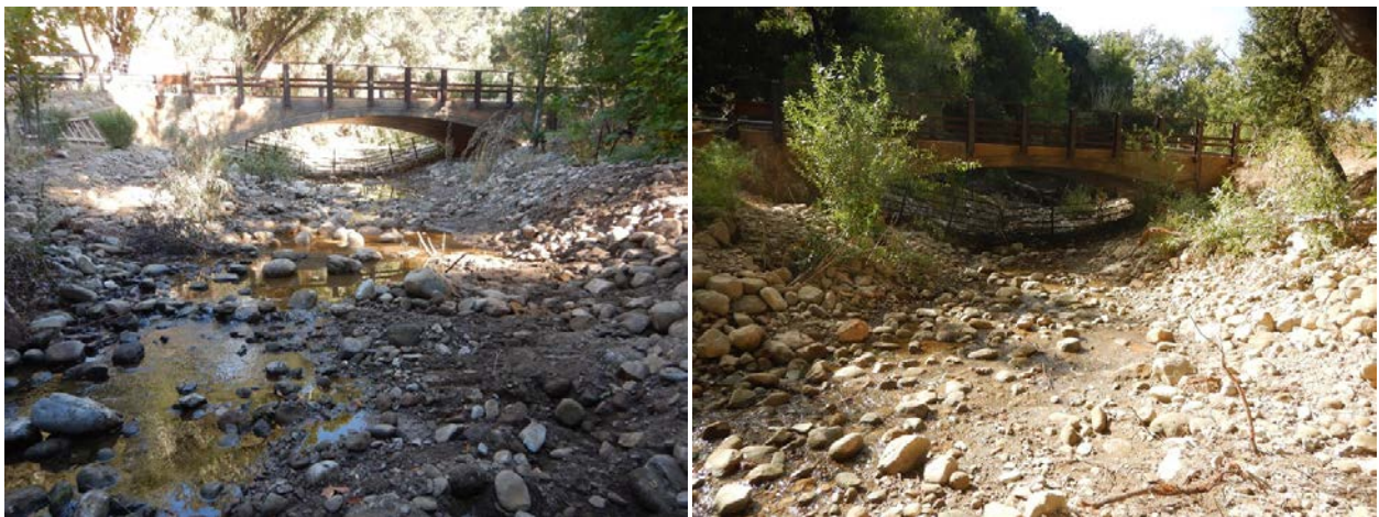
Figure 3: Quiota Creek Crossing 5 completed project.
