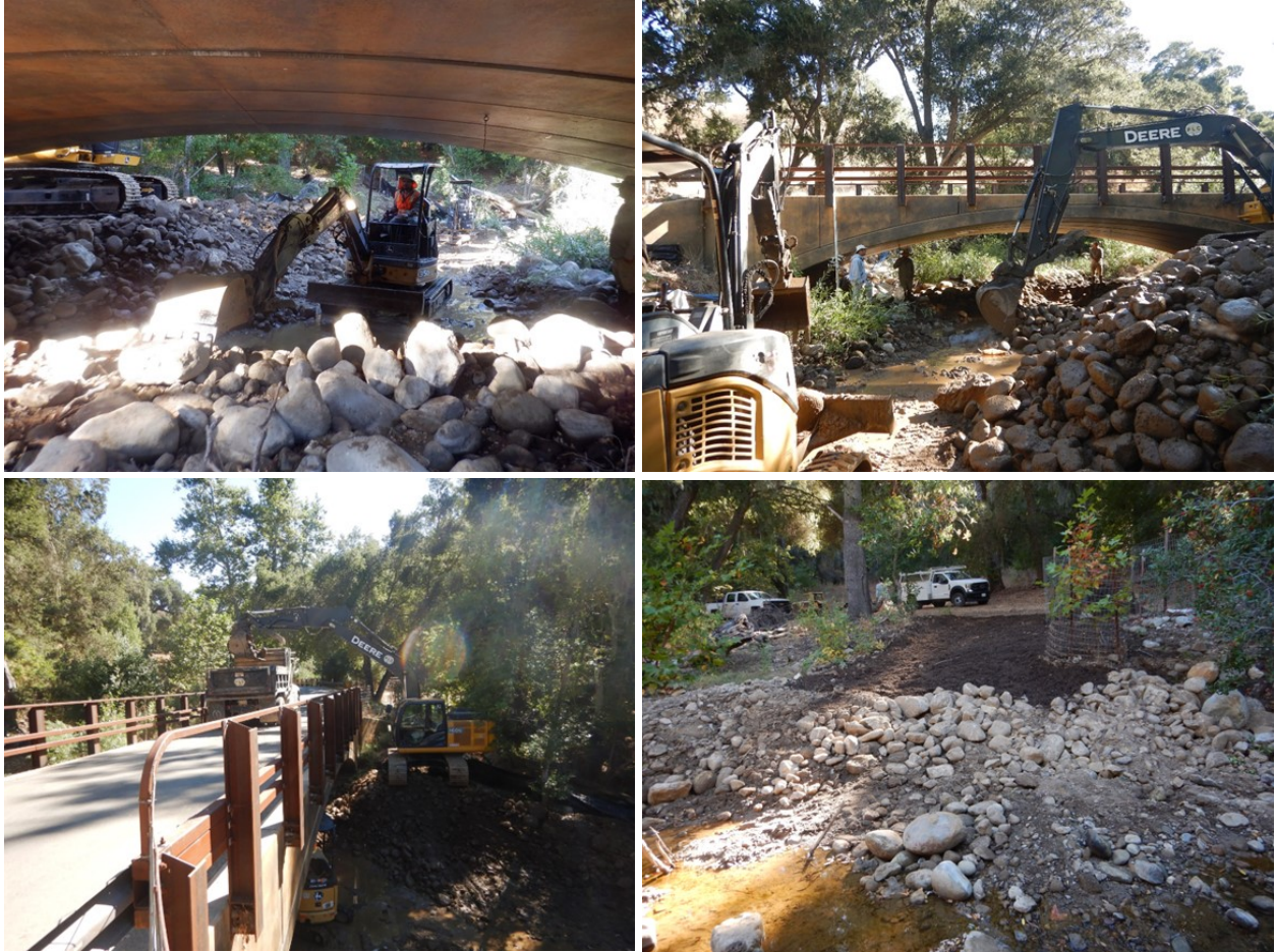
Figure 2: Quiota Creek Crossing 5 construction.
