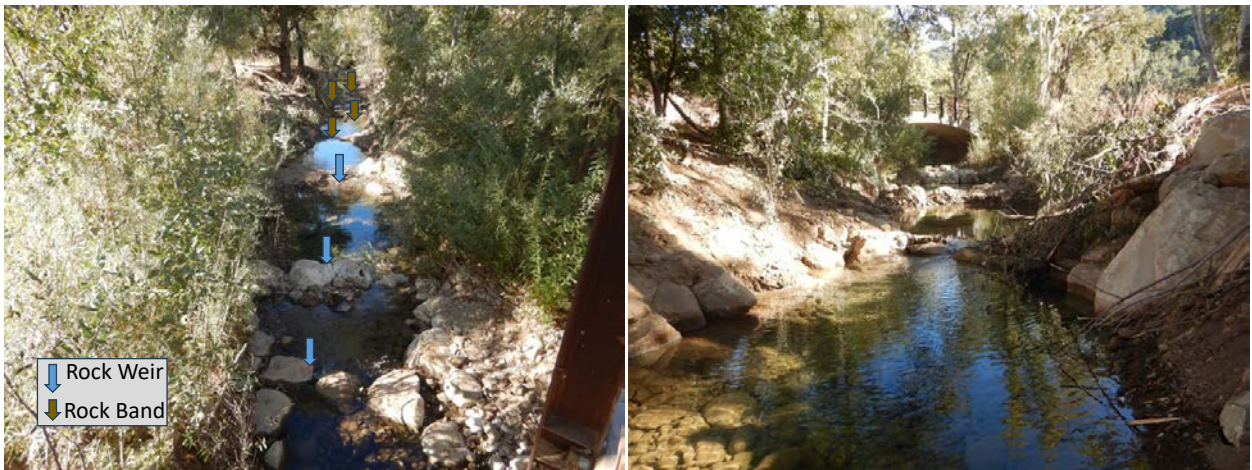
Figure 6: Quiota Creek Crossing 9 completed project.
