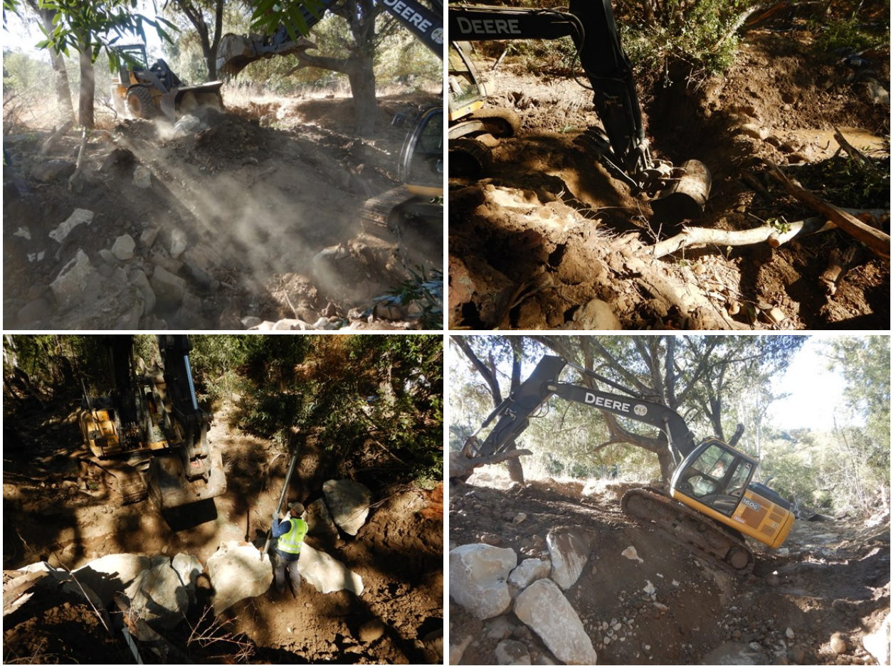
Figure 5: Quiota Creek Crossing 9 construction.
