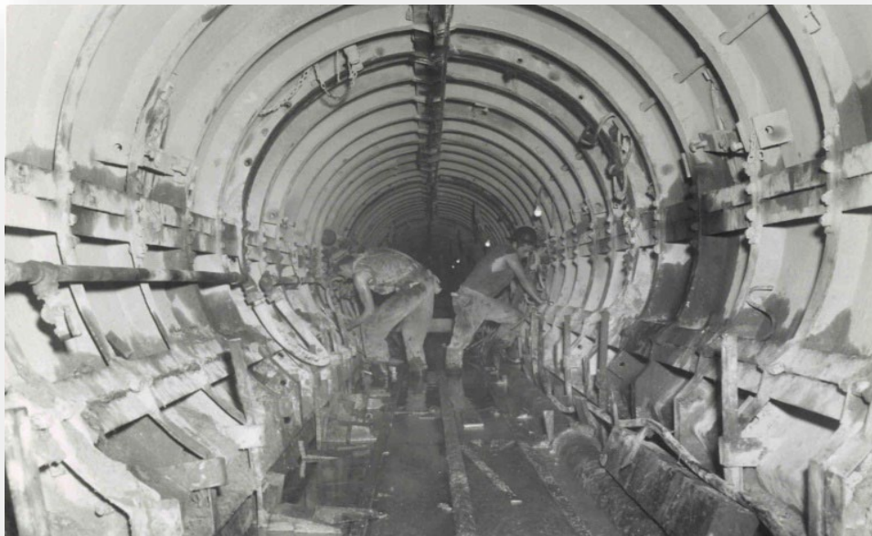
Tecolote Tunnel Construction
