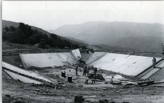
Construction of Bradbury Dam
