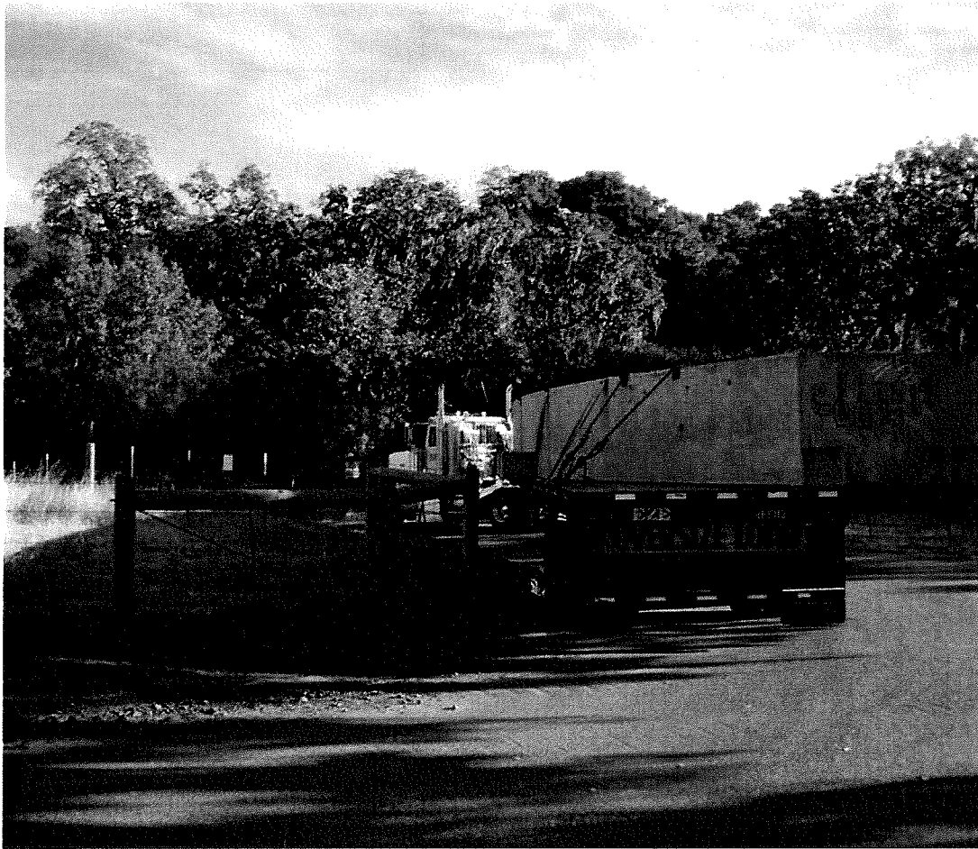
Figure 5: Transporting the bridge up Refugio Road (10/3/12).
