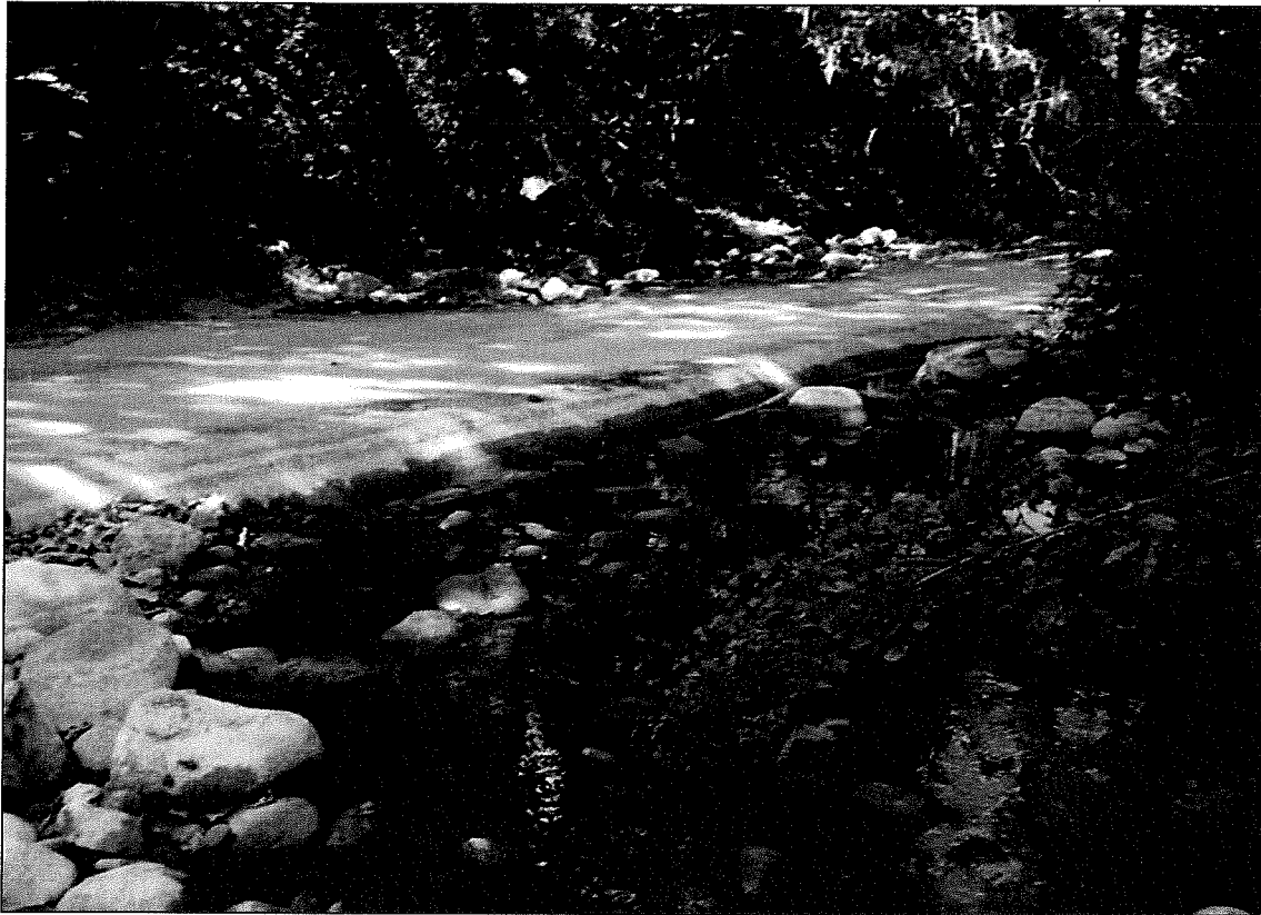
Figure 1: Quiota Creek Crossing 7, pre-project condition.
