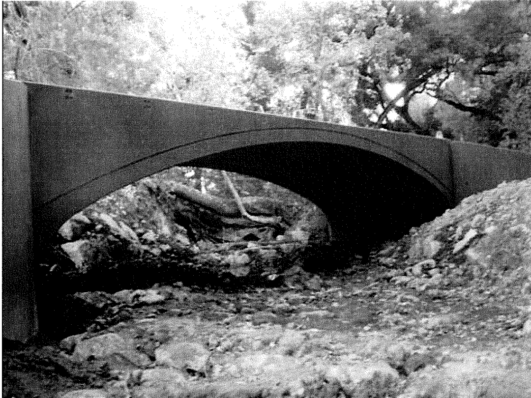
Figure 11: Painted (anti-graffiti proofing) bridge with rock weirs beneath (10/15/12).
