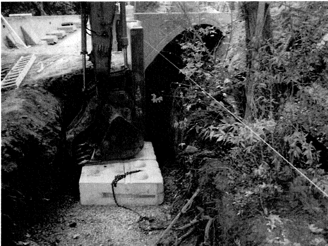
Figure 10: Block wall installation (10/15/12).
