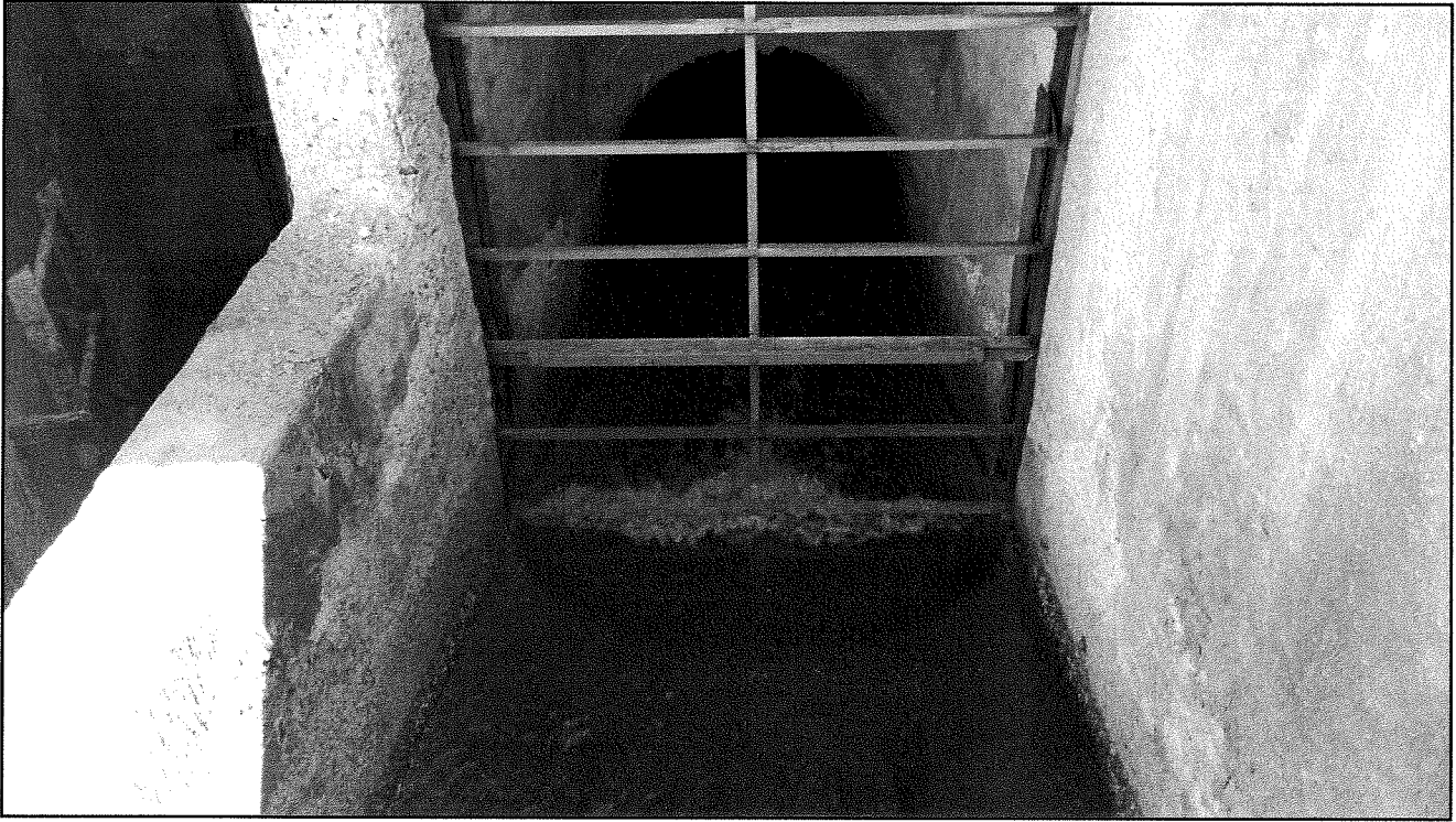
Water flowing from Junction Structure into 48" Conduit
