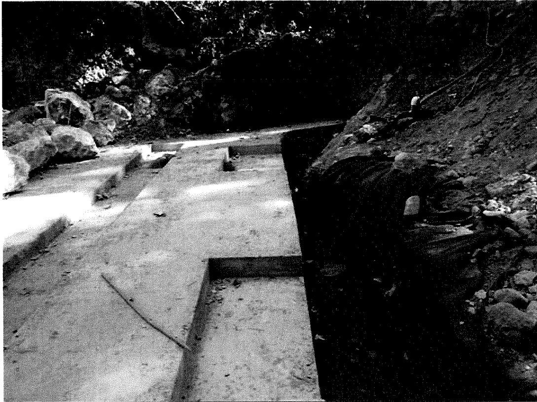
Figure 3: Completed bridge foundation (9/25/12).
