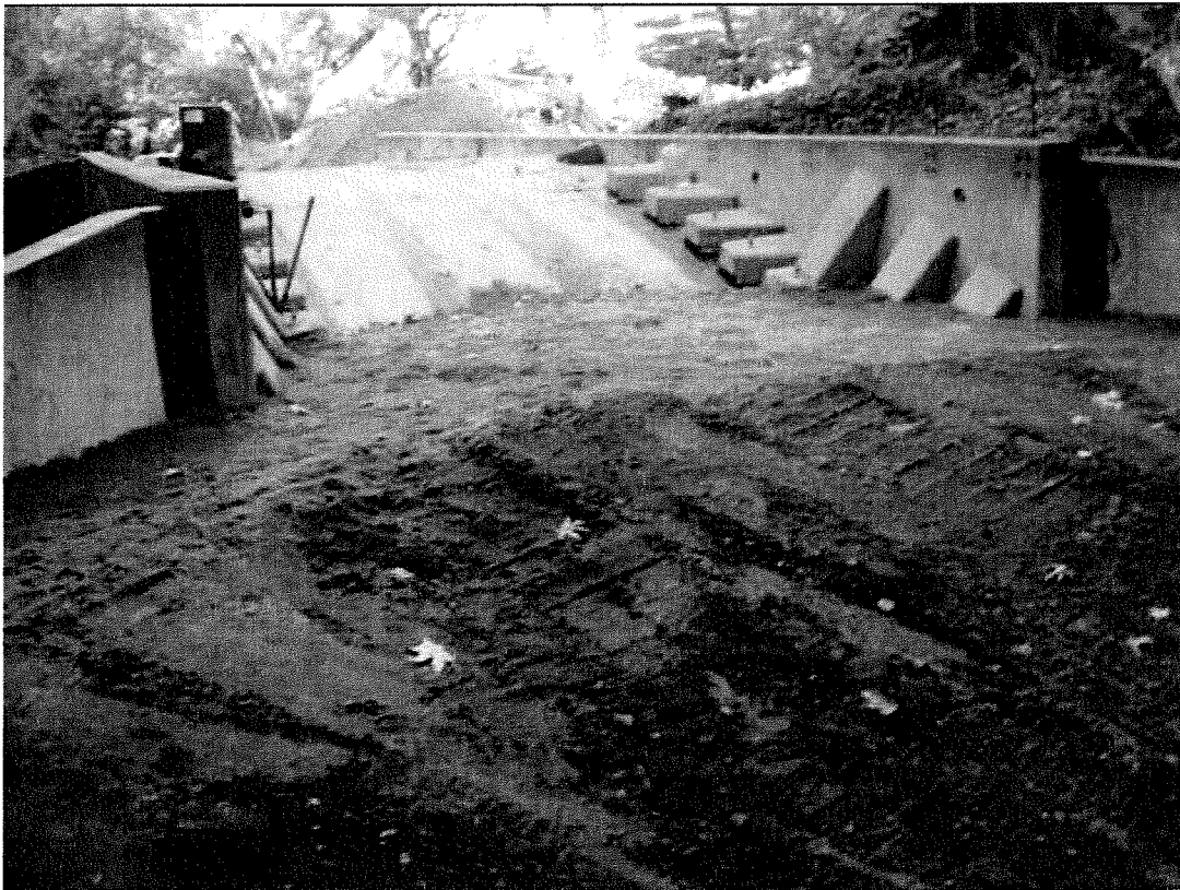
Figure 12: Backfilling the arch with 4 feet to go (10/15/12).
