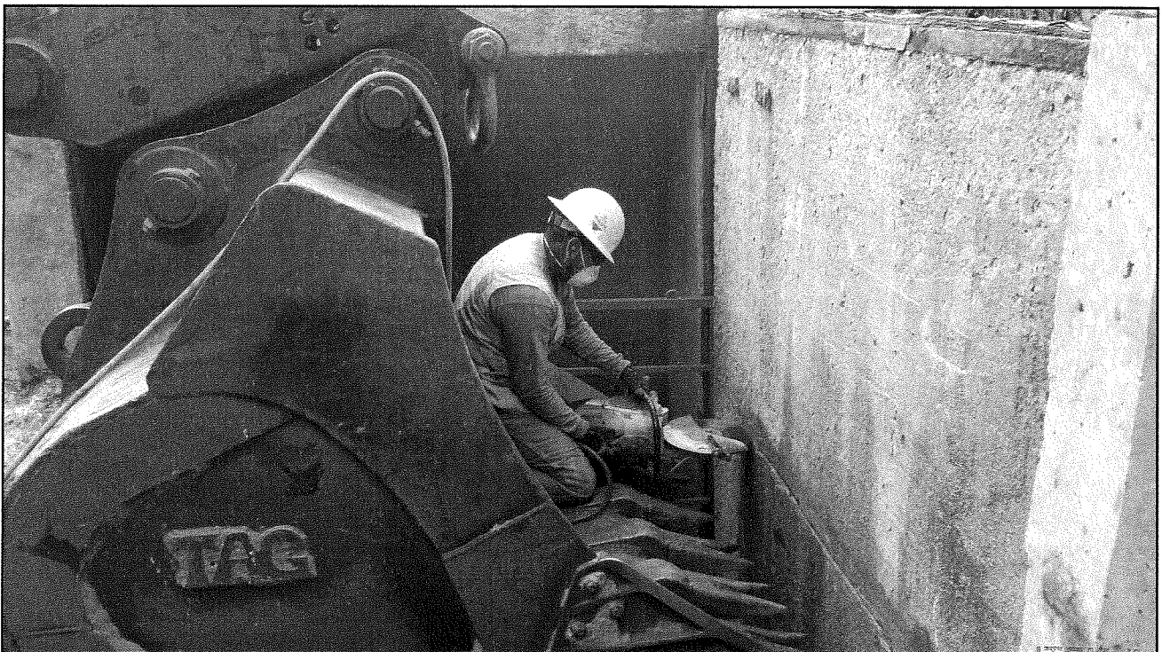
Saw cutting South Portal Junction Structure walls with diamond blade
