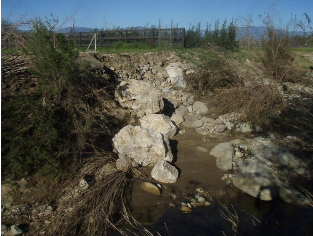
Figure 3: Rock vane at the upper end of the project showing erosion to the installed bank projection rocks (2/28/17).
