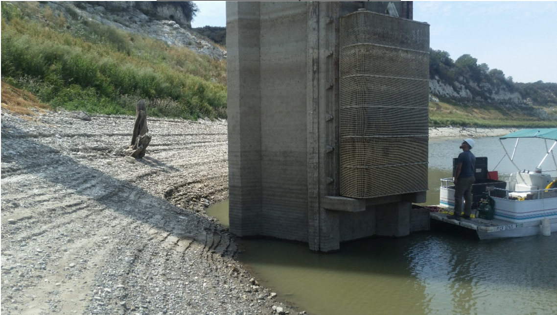
North Portal dive inspection/repairs
