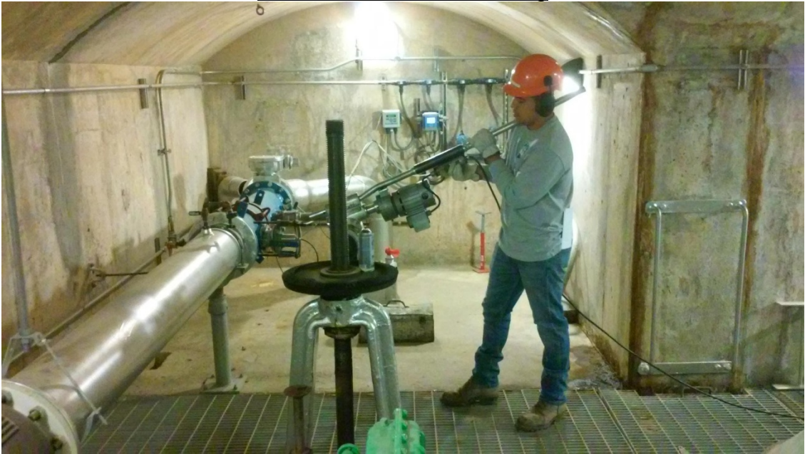
North Portal valve exercising
