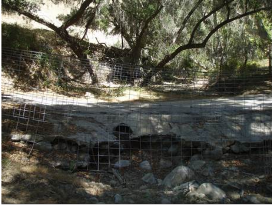
Figure 1: Pre-project condition looking upstream.
