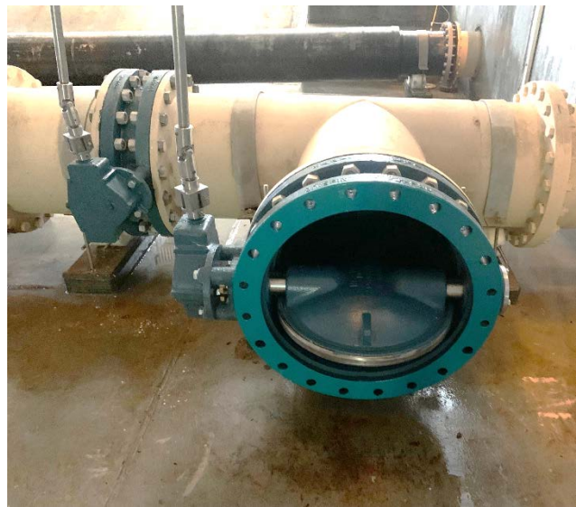
New valves operational
