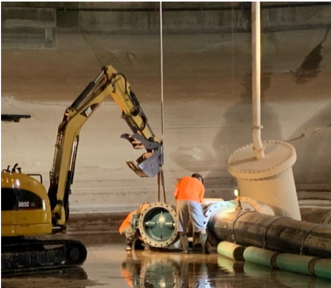
Installing new valves
