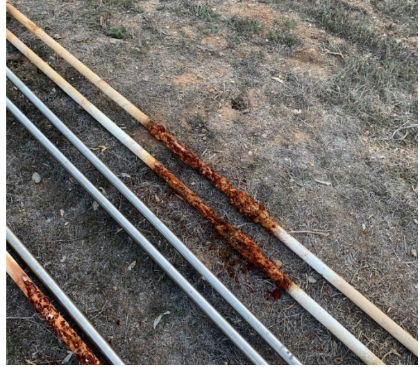
Corroded extensions compared to new extensions
