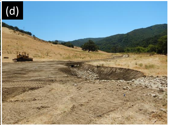
Figure 3: Construction of Basin 2 showing (a+b) basin excavation, (c) placement of inlet and outlet native cobbles, and (d) near completed condition.
