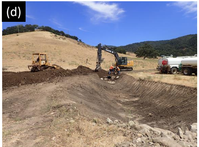
Figure 4: Ranch road culvert installation showing (a) trenching for the culvert, (b) compacting material over the culvert, (c) placement of outlet native cobbles, and (d) near final condition.
