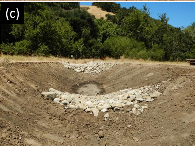
Figure 3: Construction of Basin 2 showing (a+b) basin excavation, (c) placement of inlet and outlet native cobbles, and (d) near completed condition.
