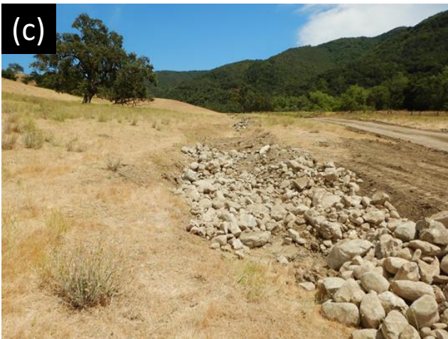
Figure 5: Ranch road drainage treatment showing (a) grading of the road, (b) road side drainage ditch grading, (c) native cobble bar placement within the drainage ditch and (d) completed condition with mulch.
