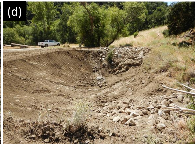
Figure 2: Construction of Basin 1 showing (a) basin excavation, (b+c) placement of inlet and outlet native cobbles, and (d) near completed condition.
