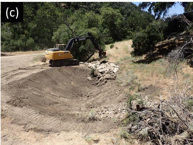
Figure 2: Construction of Basin 1 showing (a) basin excavation, (b+c) placement of inlet and outlet native cobbles, and (d) near completed condition.
