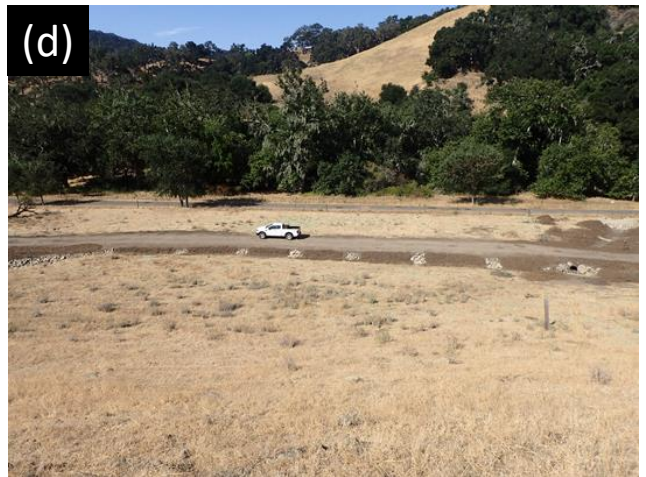
Figure 5: Ranch road drainage treatment showing (a) grading of the road, (b) road side drainage ditch grading, (c) native cobble bar placement within the drainage ditch and (d) completed condition with mulch.
