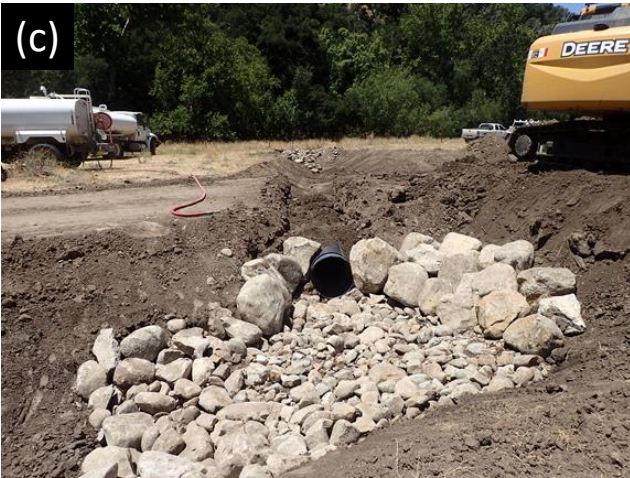
Figure 4: Ranch road culvert installation showing (a) trenching for the culvert, (b) compacting material over the culvert, (c) placement of outlet native cobbles, and (d) near final condition.
