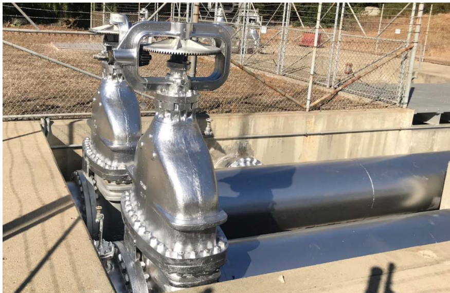
Lauro Control Station after painting
