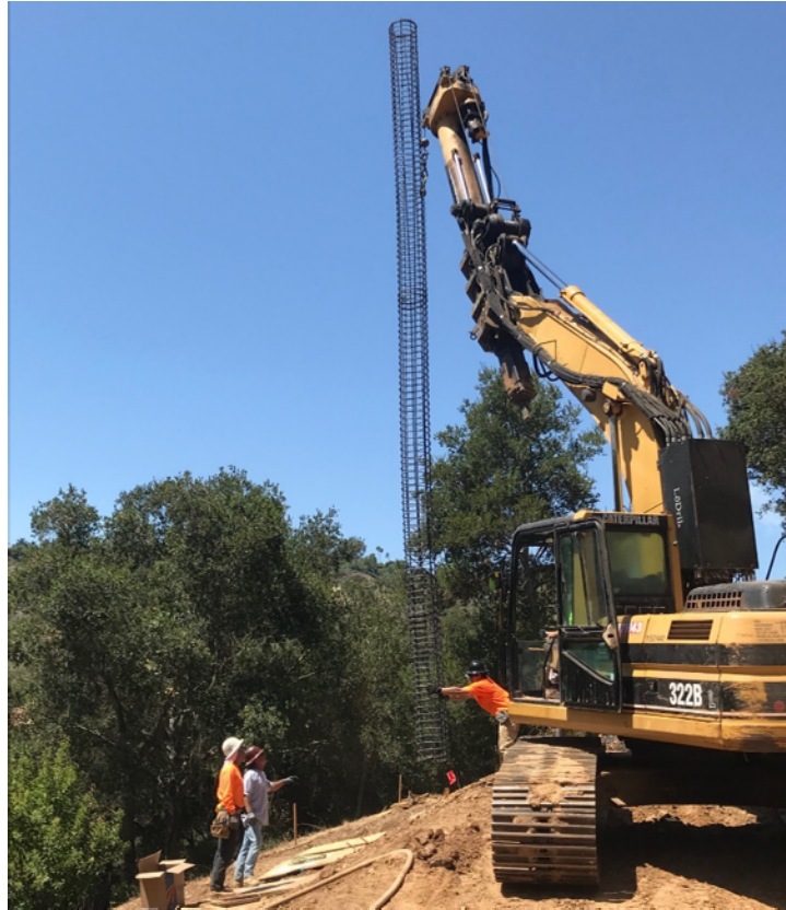
Installation of rebar cages prior to pouring concrete for reinforced caissons
