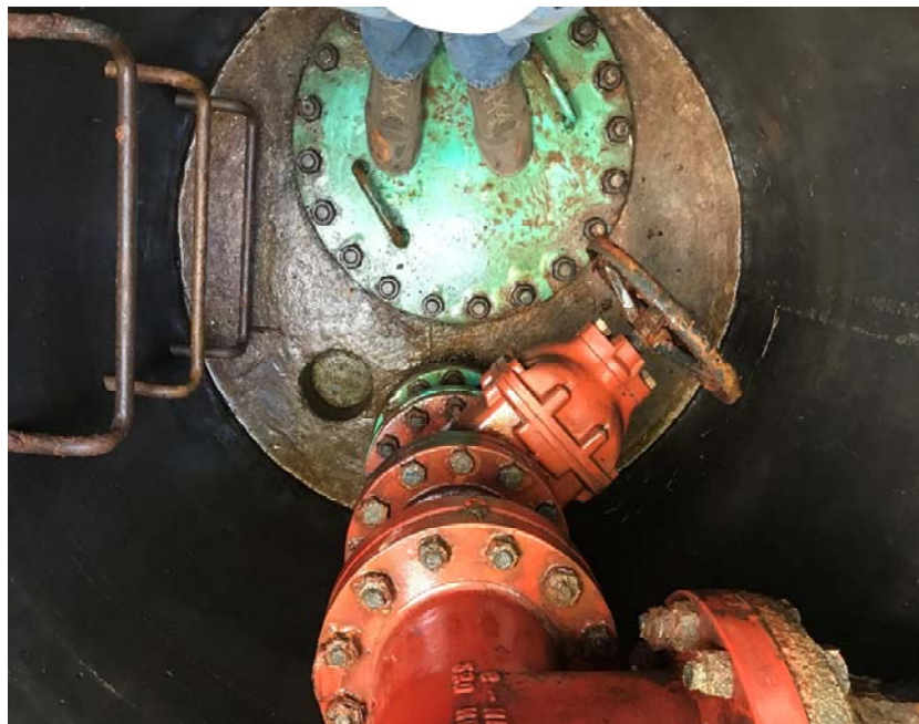
Inside of blowoff structure after cleaning
