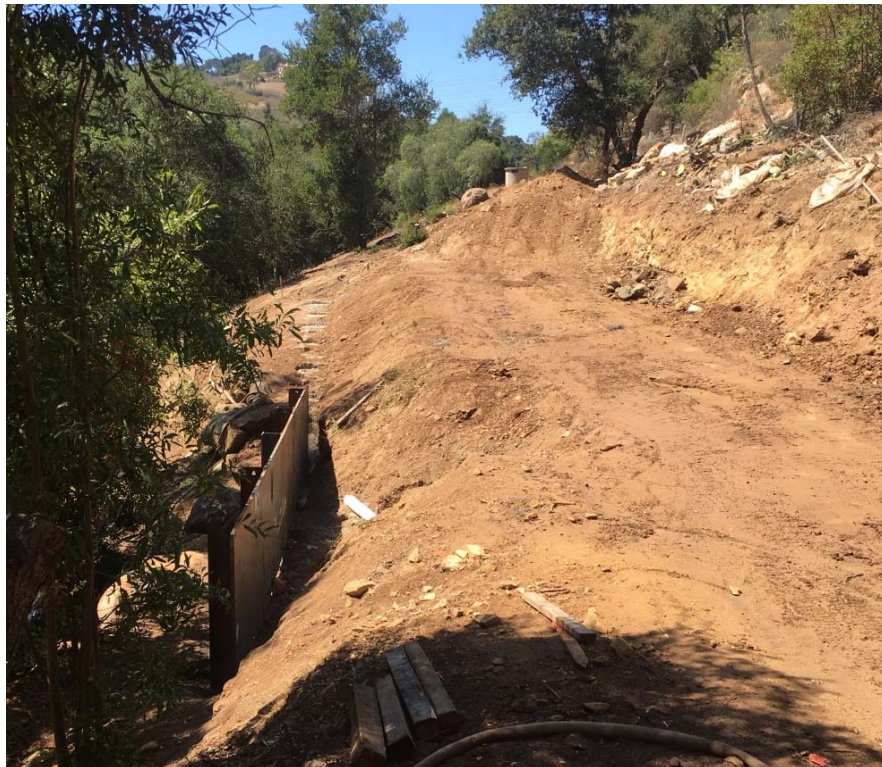
Completed 70-foot long reinforced caisson wall
