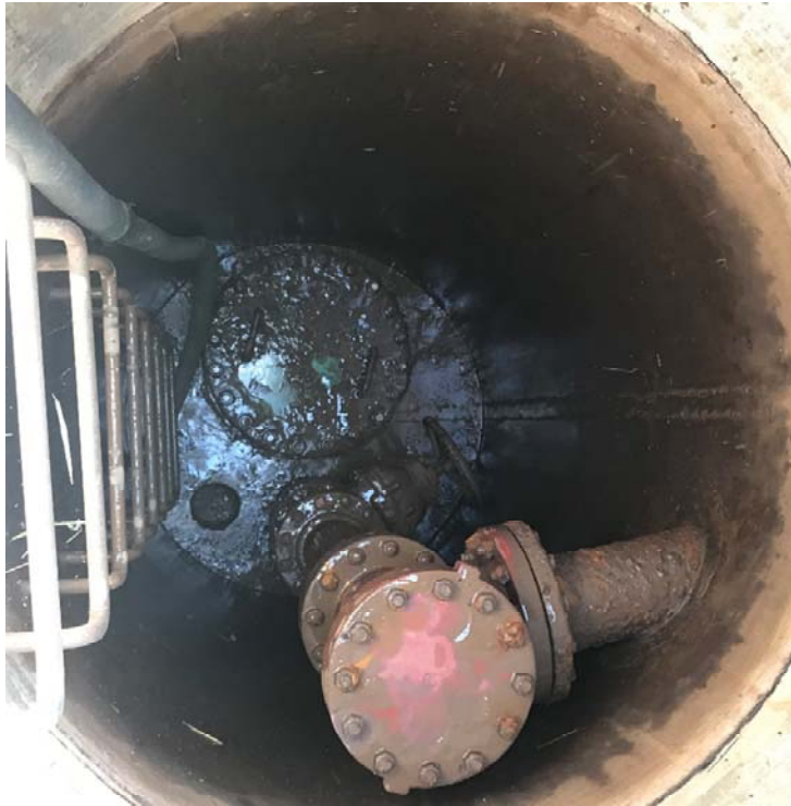
Inside of blowoff structure before cleaning
