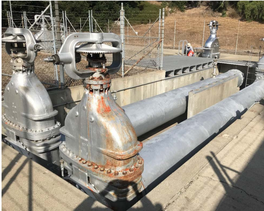
Lauro Control Station before painting
