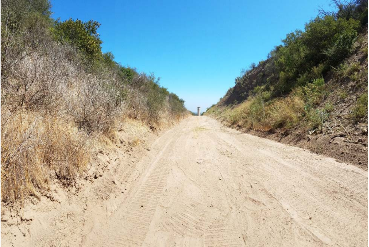
Right of Way Clearing
