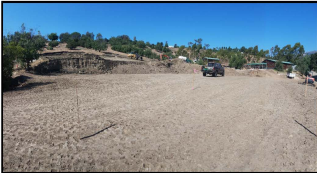
Installation of Geofoam over the South Coast Conduit to prevent overloading.
