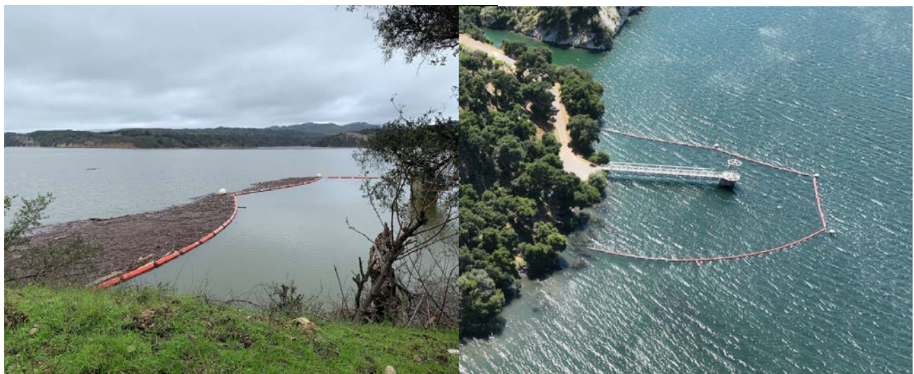
Figure 1. North Portal Log Boom keeping floating debris from reaching the Intake Tower following 2023 storms (left); Log boom limiting recreational boat access near the tower in June 2024 (right).
