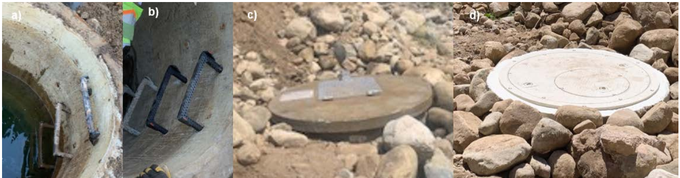
Figure 4. Toro Canyon Blowoff Vault Repairs and Mitigation
