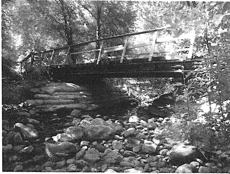
Figure 6: Quiota Creek on Refugio Road showing upstream view of Crossing 8.
