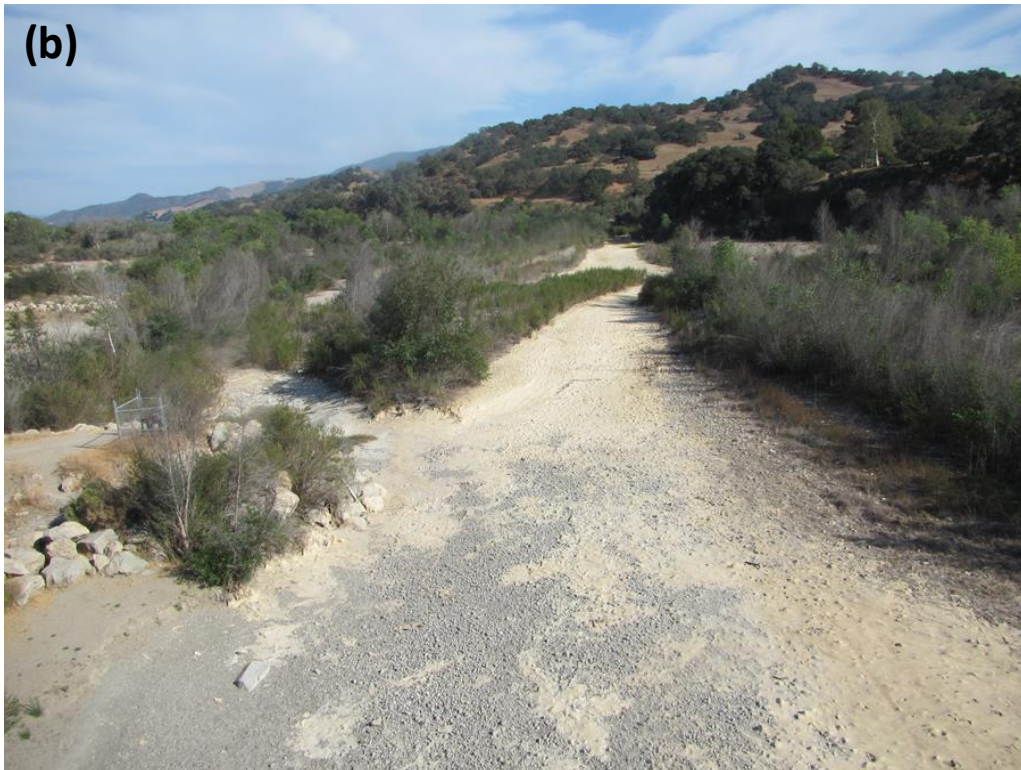
Figure 32: Photo point (M-14) collected at Alisal Bridge looking upstream in a) May 2005, and b) September 2016. Note all the dead riparian vegetation.
