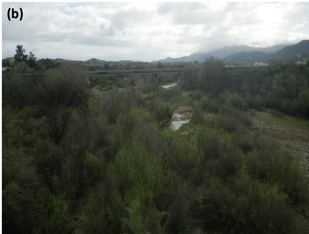
Figure 33: Photo point (M-19) collected at Avenue of the Flags Bridge looking upstream in (a) May 2005, and (b) March 2016.
