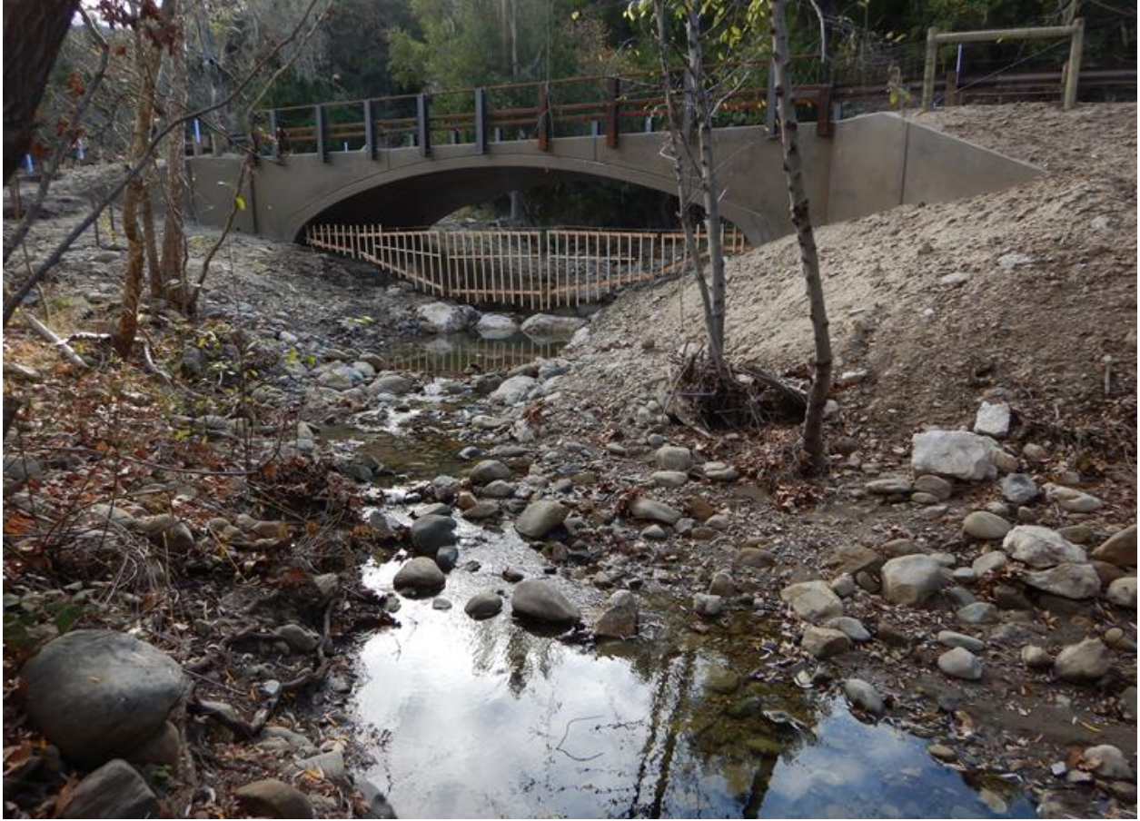
Figure 3: Completed project with streamflow.
