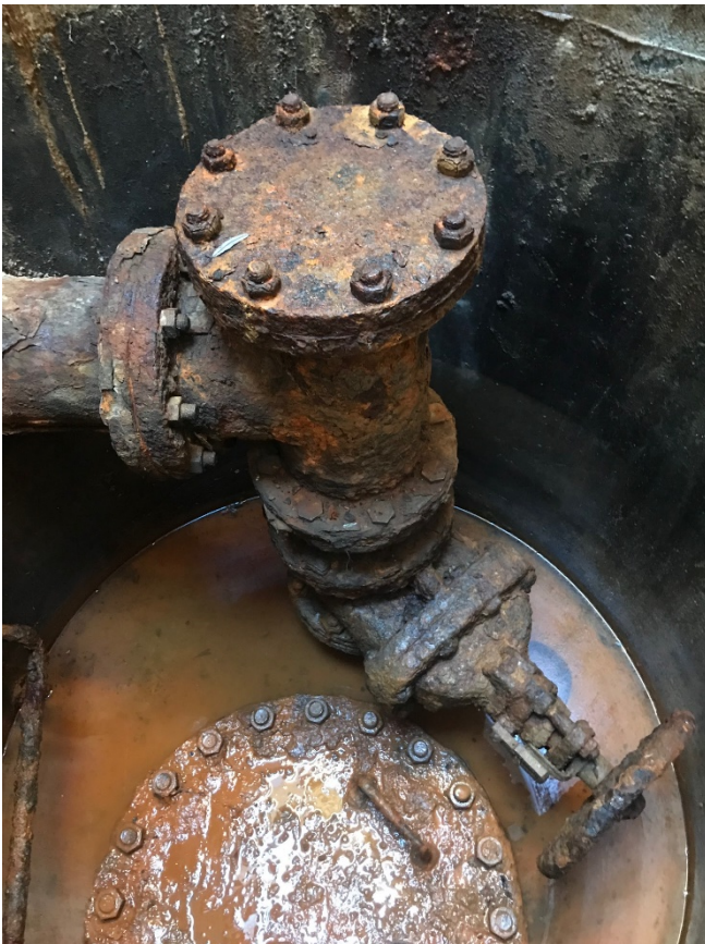
Blowoff Station 552+45 before rehabilitation work
