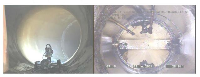
**Figure 3**. Goleta West Conduit – Video Camera Inspection – Inspection camera (left) and bottom of Glen Anne Turnout - Butterfly Valve #5. Mortar lining in good condition and tight seal achieved with Butterfly Valve #5.
