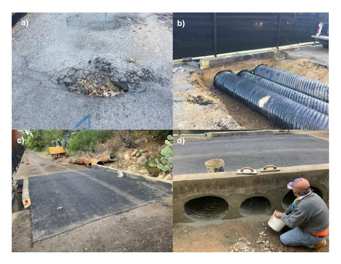
**Figure 4.** Sheffield Control Station Access Road Culvert Repair - a) Sinkhole starting to form in roadway over the South Coast Conduit alignment due to collapse culvert; b) new polymer-coated corrugated steel culverts that should better resist future corrosion; c) slurried and paved portion of the access road over the new culverts. *Note:* the rusted condition of the corroded culverts in the background; and d) repair of headwall.
