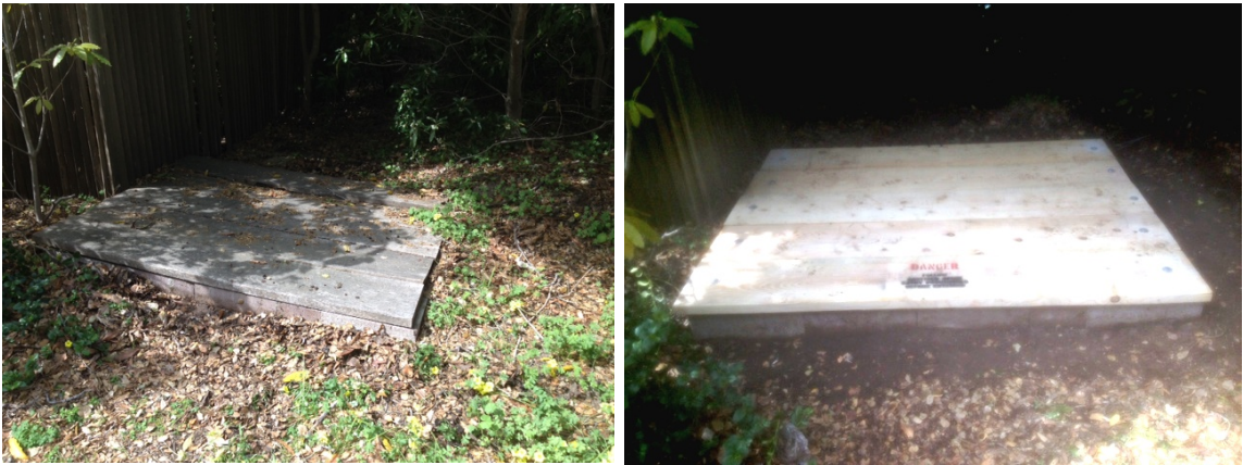
Hot springs lateral structure cover replacement
