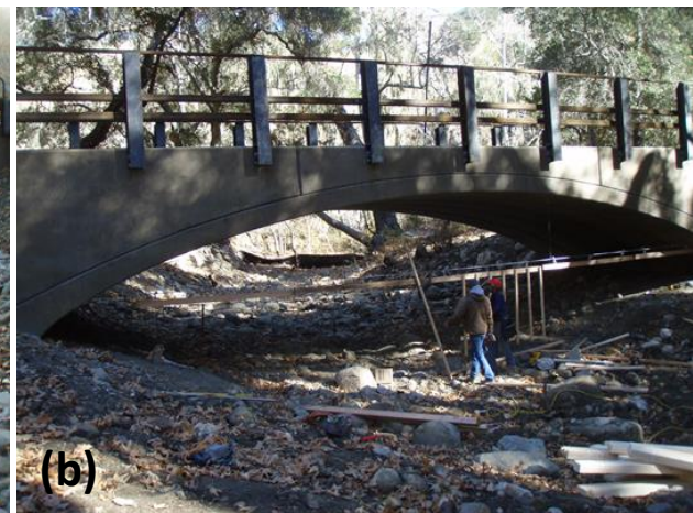
Figure 8: Completed (a) instream work looking downstream and (b) bridge-rail with picket cattle fencing being installed below the bridge.
