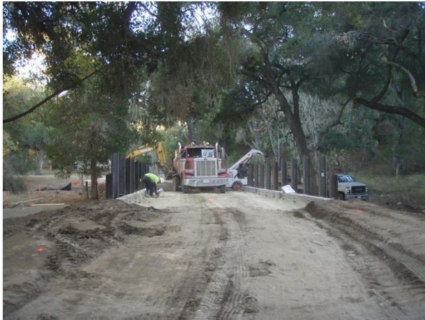
Figure 1: Installing road base and bridge-rail posts.
