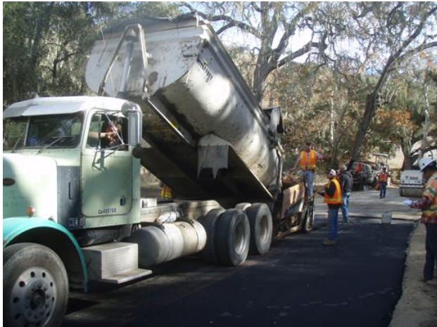
Figure 4: Paving Refugio Road through the project site.
