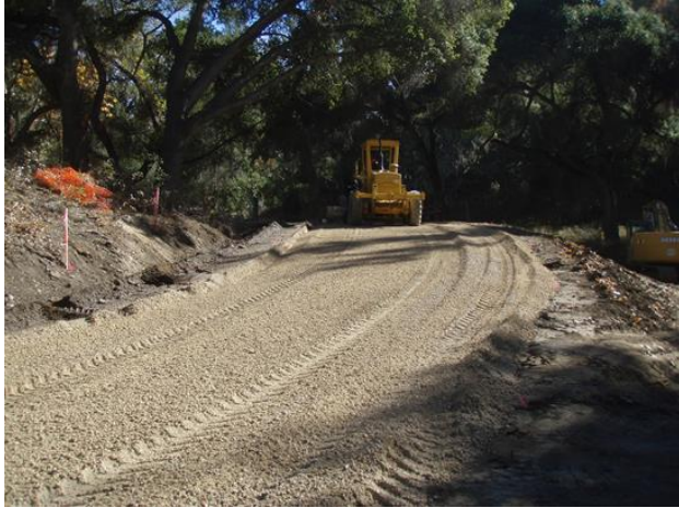
Figure 3: Grading and compacting the road base.
