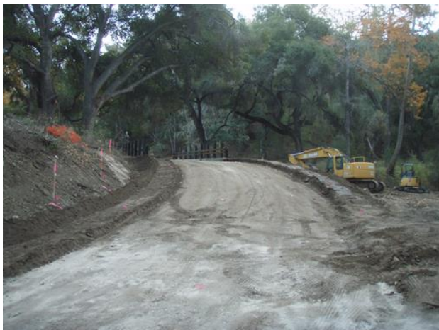
Figure 2: Installation of the road embankments and road base.
