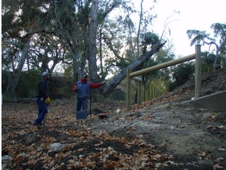
Figure 6: Installation of property fencing.
