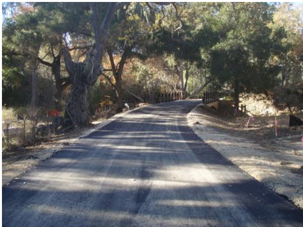
Figure 5: Completed paving and guardrail installation.
