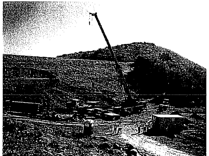
Lauro Dam Construction Project
