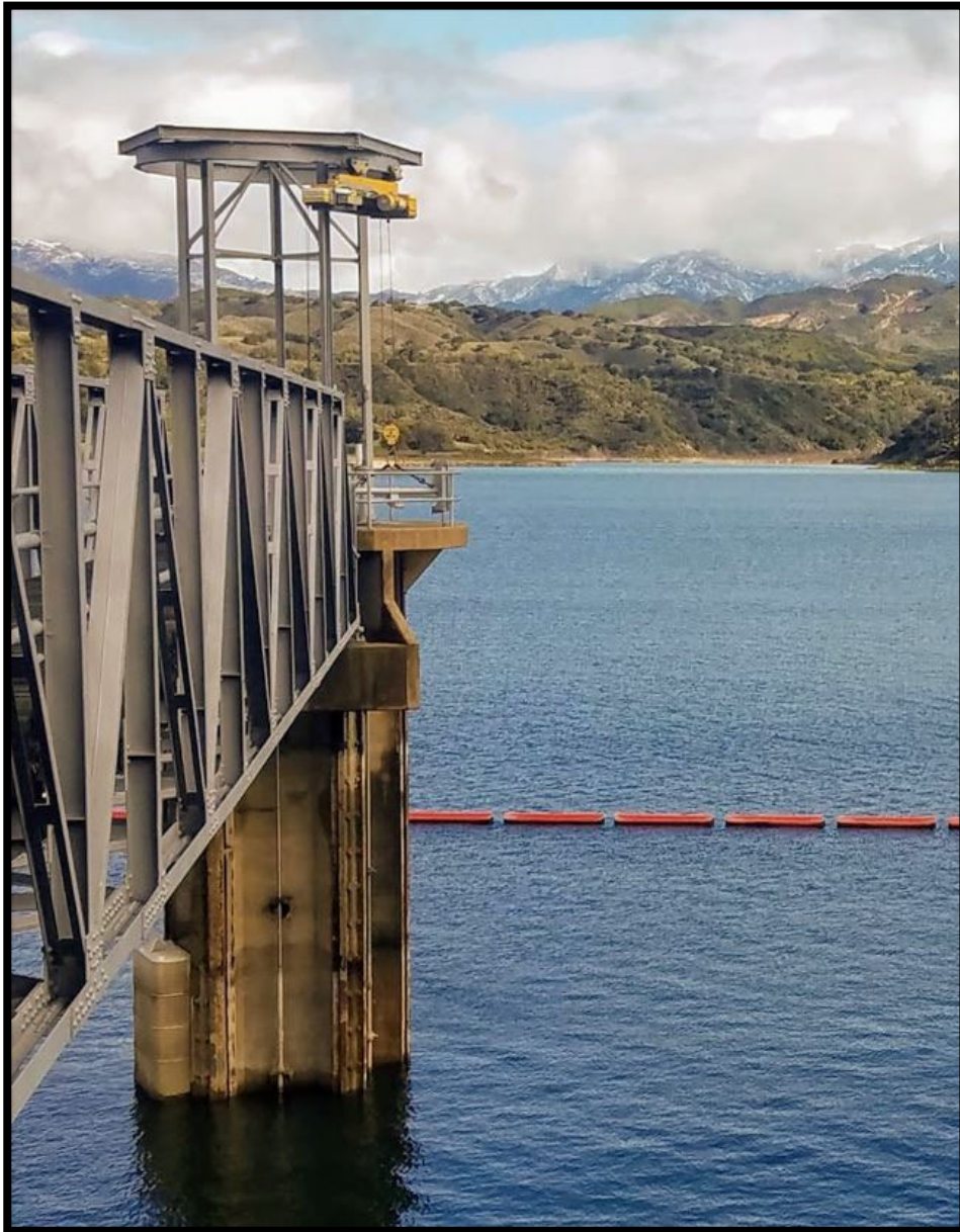
Lake Cachuma, North Portal Intake Tower
