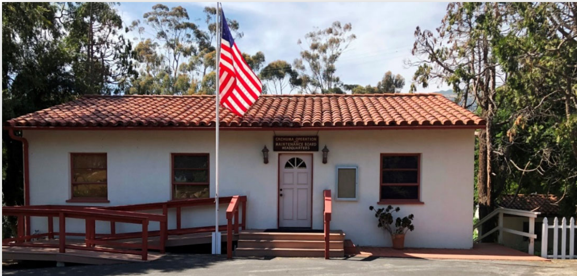
Cachuma Operation and Maintenance Board Meeting Room
