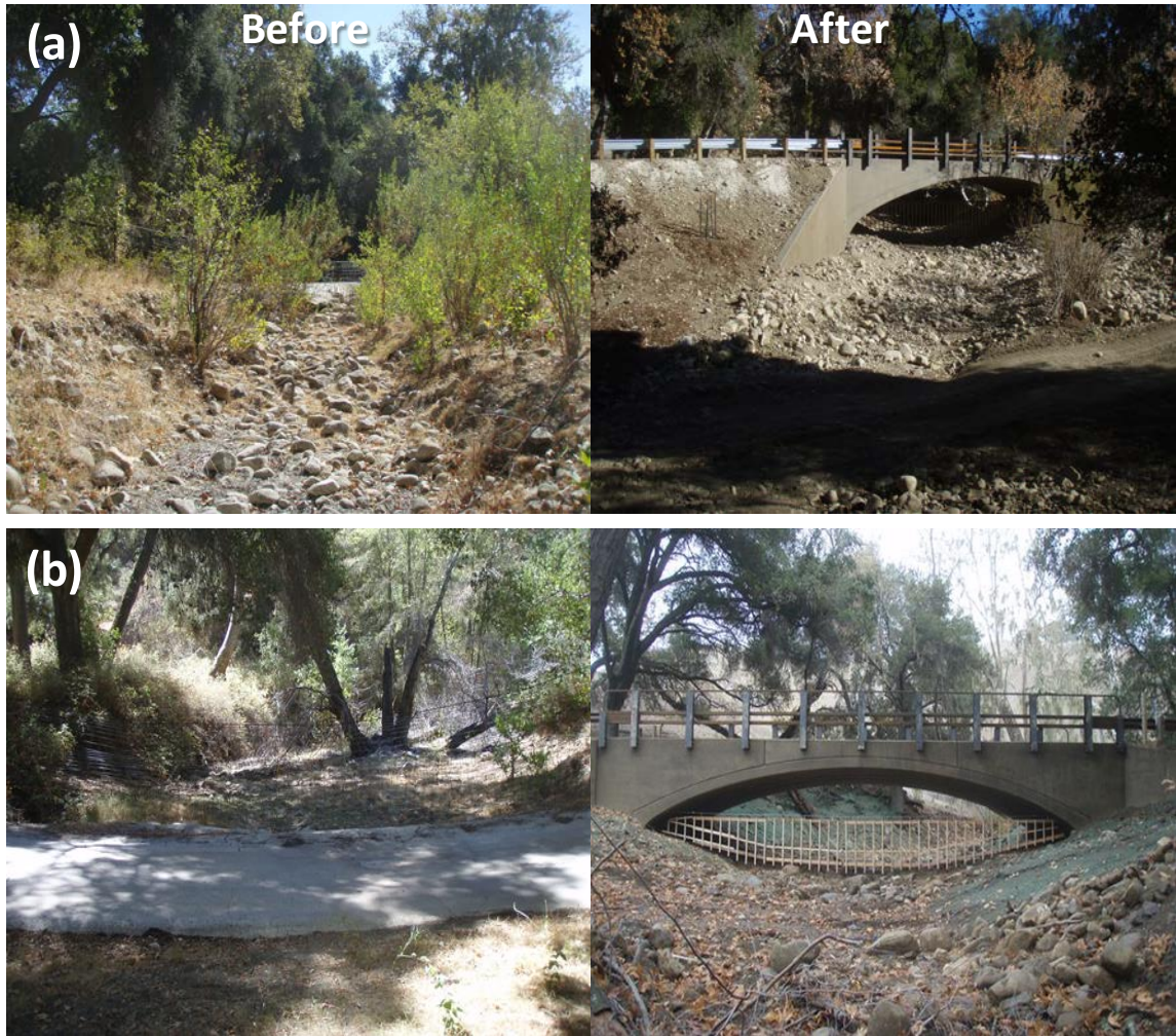
Figure 68: Fish passage and habitat restoration at (a) Quiota Creek Crossing 1 (in 2014) and (b) Quiota Creek Crossing 3 (in 2015).
