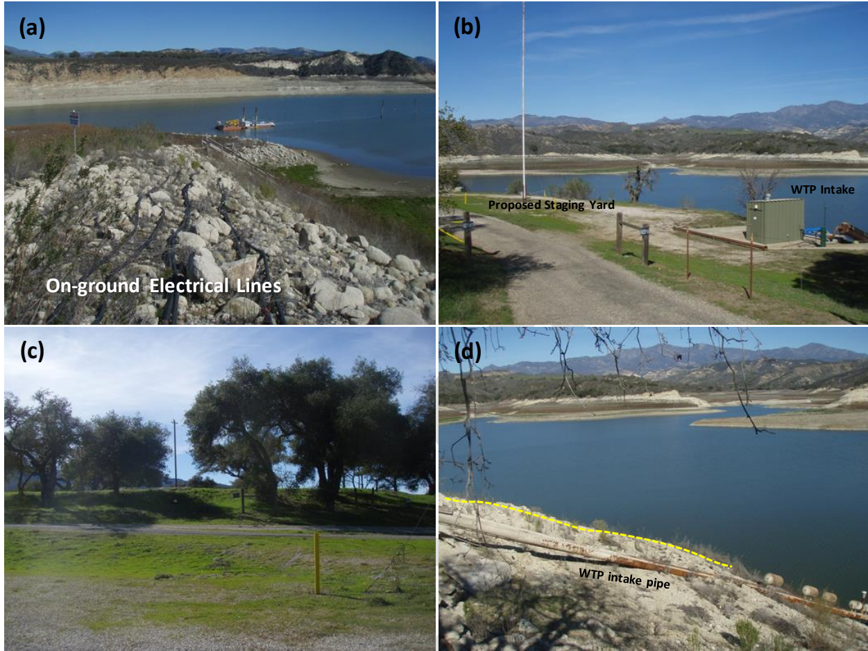
Figure 9: Staging Yard and electrical line layout specifically (a) current electrical lines laid on the bank down to the Pumping Barge in the distance at Location 1, (b) proposed Staging Yard at Location 2 next to the WTP intake all within an area closed to the public, (c) position of the proposed new PG&E drop pole to the existing PG&E power pole, and (d) layout of the electrical line in yellow from the Staging Yard to the Pumping Barge just to the north of the WTP intake pipe.
