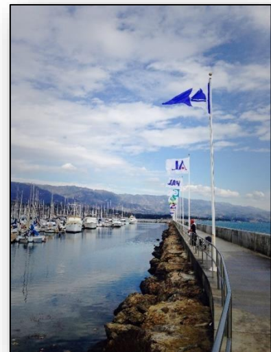
Breakwater at Santa Barbara Harbor
