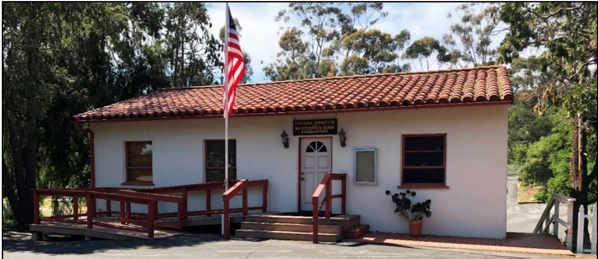
COMB Board Room
