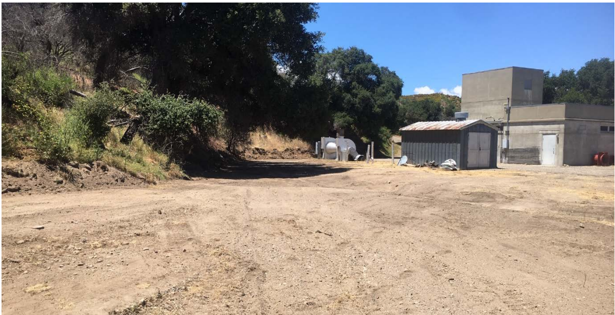
Defensible space and drainage maintenance around the North Portal Control Building
