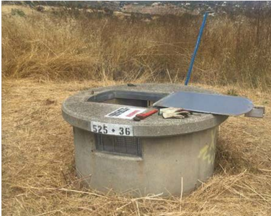
Vegetation cleared around structure 525+36
