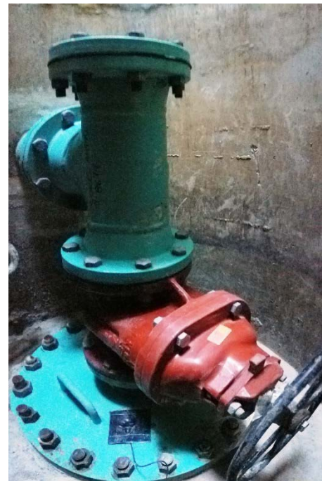
Replaced outlet, valve and piping in a blowoff structure
