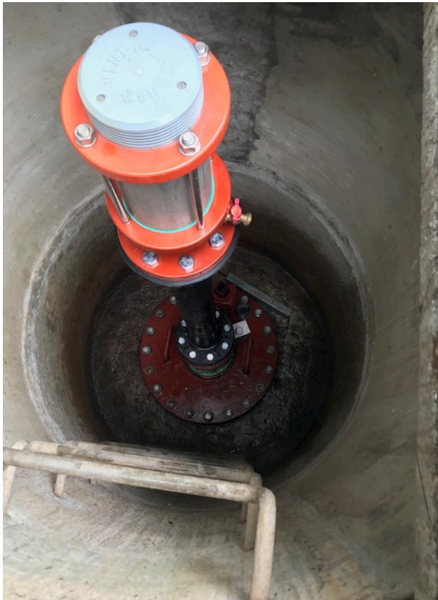
Raised air vent at structure 495+30
