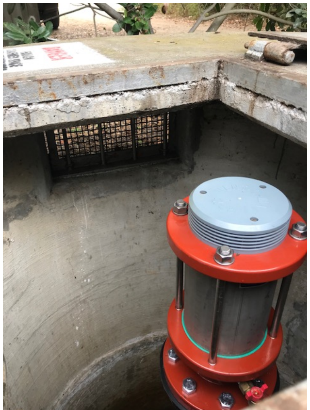
Raised air vent at structure 495+30
