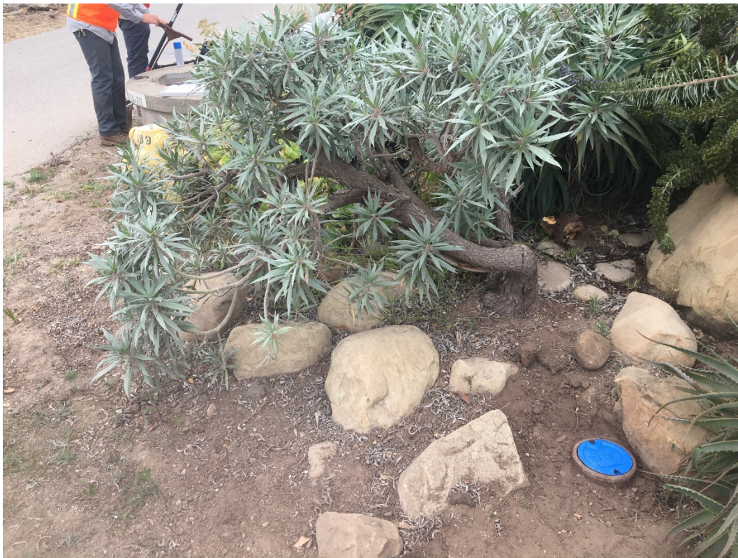
Located buried valve at Lateral 13L with metal detector
