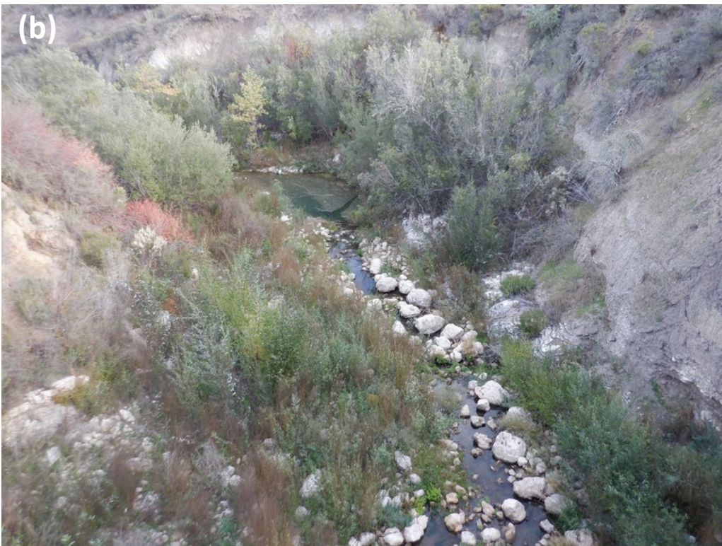
Figure 65: Photo point (T-39) collected at Salsipuedes Creek at Hwy 1 Bridge in May 2005 and (b) October 2022 (Post CalTrans Hwy 1 Bridge Replacement Project).
