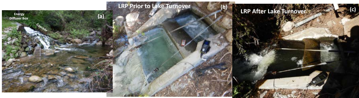
Figure 105: Hilton Creek (a) release point configuration showing energy diffusion box and cascade, (b) LRP prior to lake turnover, and (c) LRP after lake turnover.
