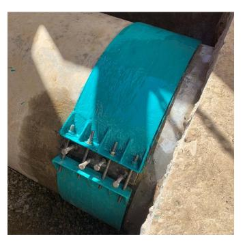
Installation of Custom-fabricated repair clamp for outflow pipeline
