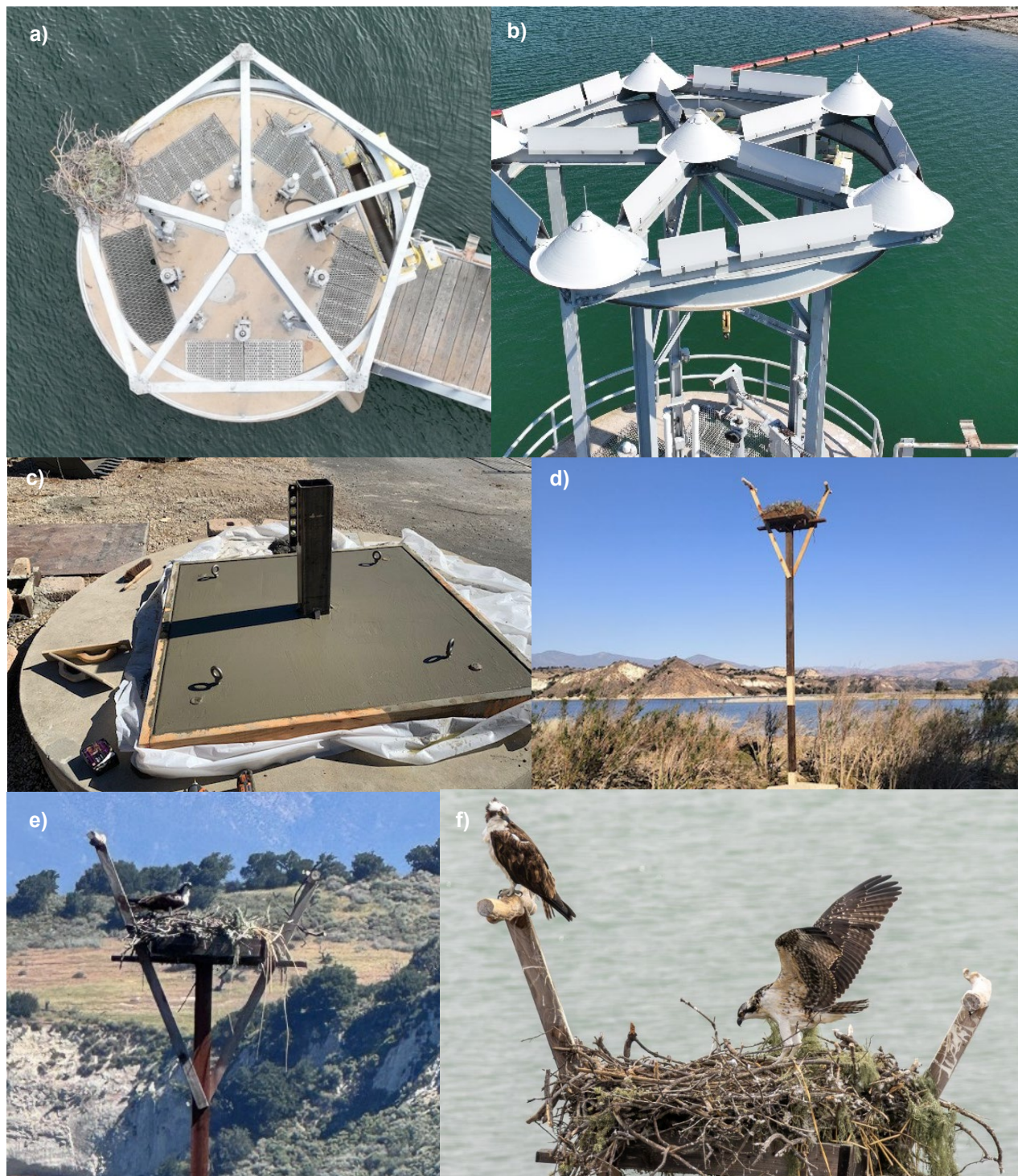
Figure 2. a) Osprey nest on the Intake tower confirmed to be inactive in Fall 2025; b) nest diverters installed on the intake tower in Fall 2025; c, d) mobile nesting platform constructed in Fall 2024; e) osprey pair building nest on platform in March 2026; f) osprey nestling testing its wings 7/7/27 (courtesy Spencer Seale).
