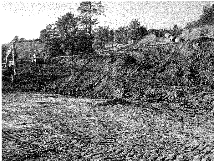
Picture 3 – Access Improvement progress
