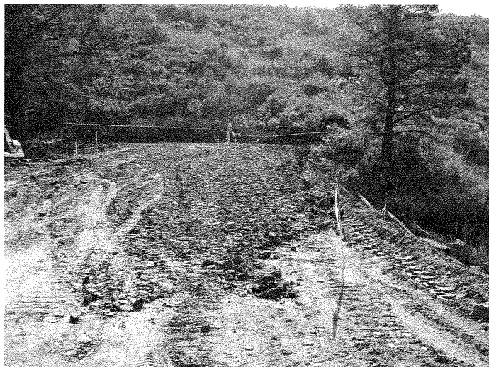
Picture 1 – Final Grading of Debris Dam
