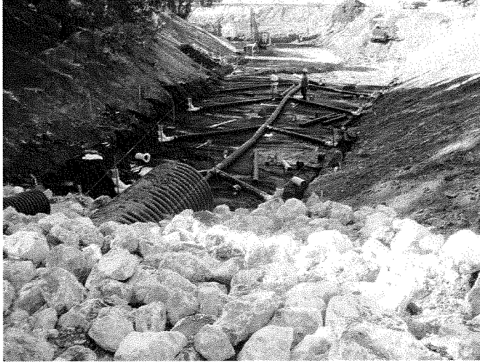
Picture 2 – Subdrain installation
