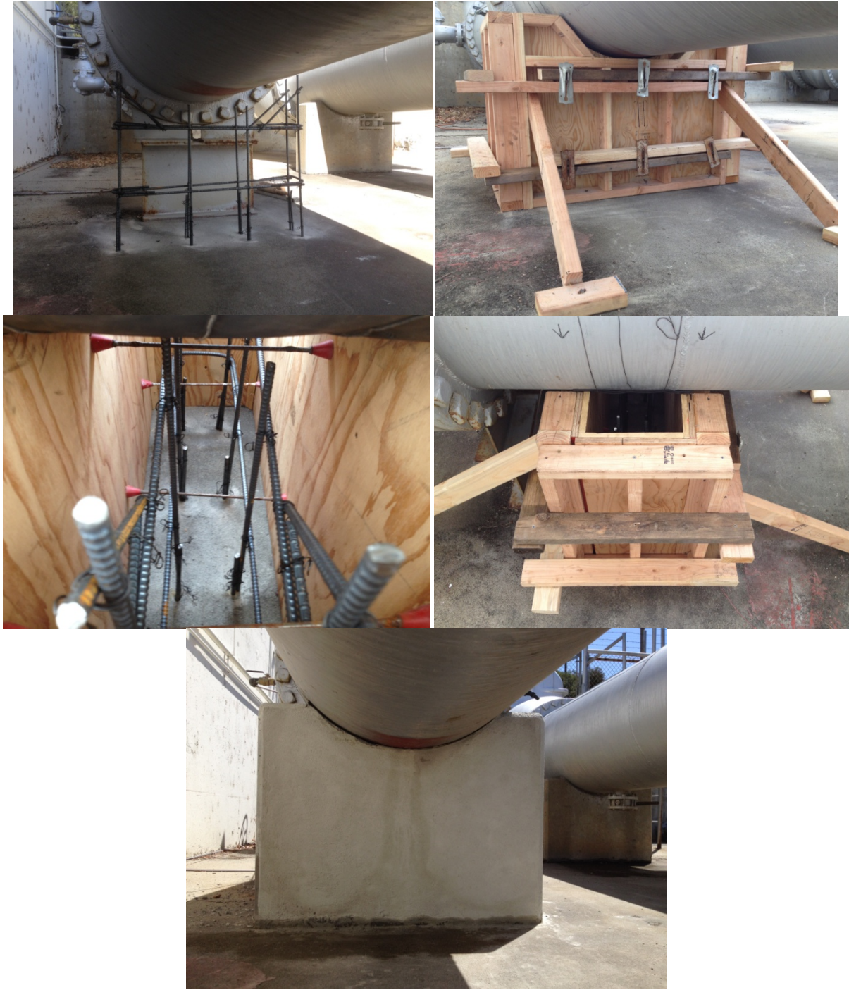
Installed concrete pipe support (before & after)
