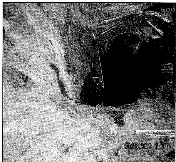
Excavating down to bed rock or firm native material
