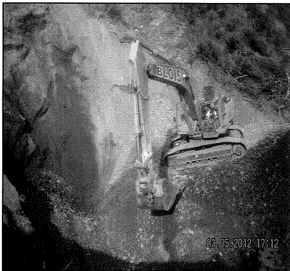
Excavating down to bed rock or firm native material
