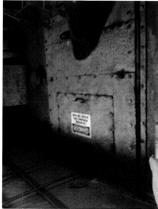
Replacing Bolts on Hatch at North Portal
