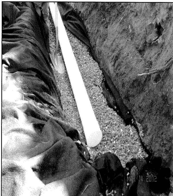
Drain pipe installation
