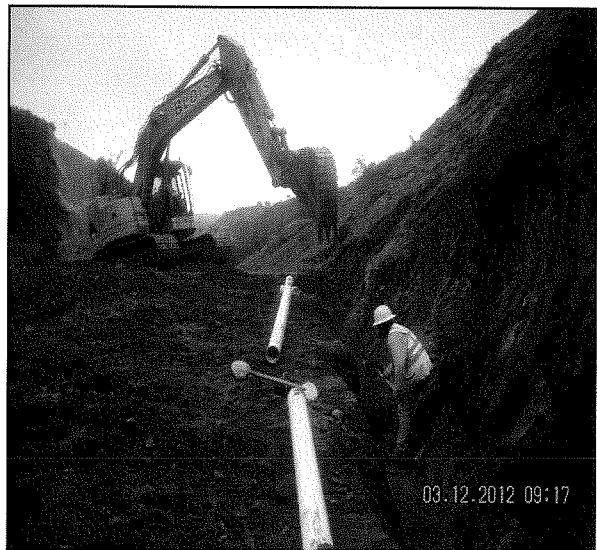
Perforated pipe is installed to carry out any water trapped between the existing slope and constructed fill. Pipe is backfilled with drain rock and wrapped in filter fabric to keep soil from clogging the holes.
