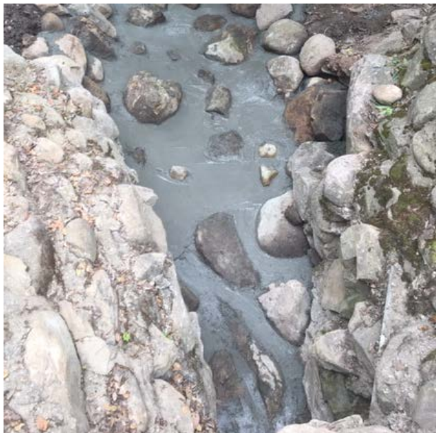
Rock and concrete channel placed over 6" reinforced concrete cap on SCC
