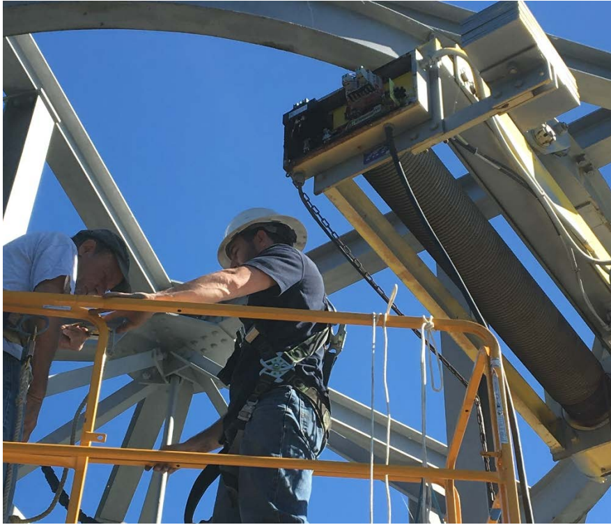
North Portal Intake Tower hoist electrical transformer replacement
