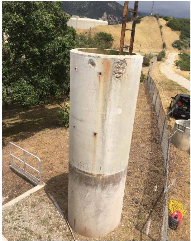
Top vault section and lid removed
