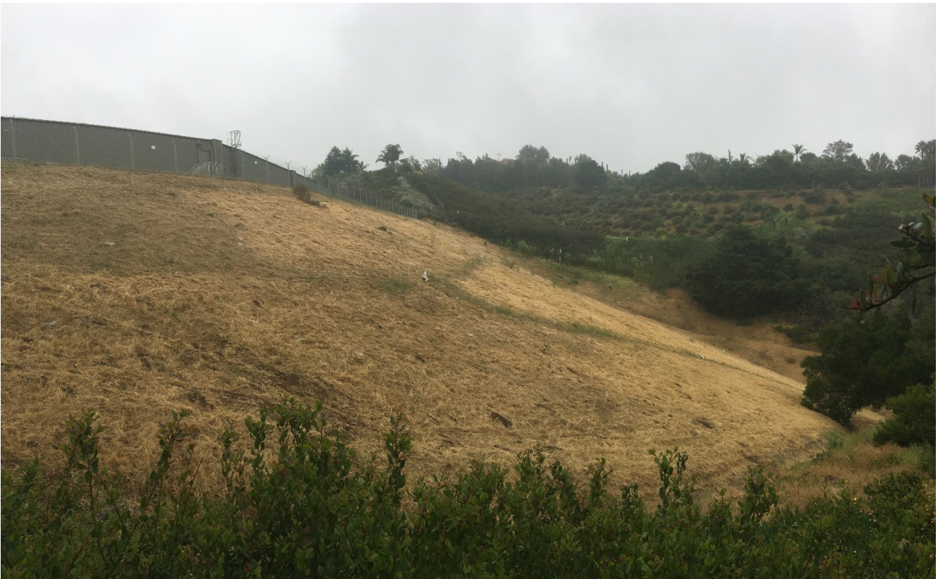
Ortega Dam face after weed abatement
