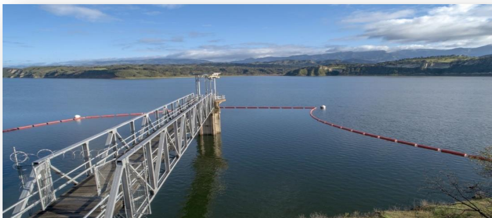
North Portal Intake Tower – March, 2019 (Photo Credit: SB County Public Works)
