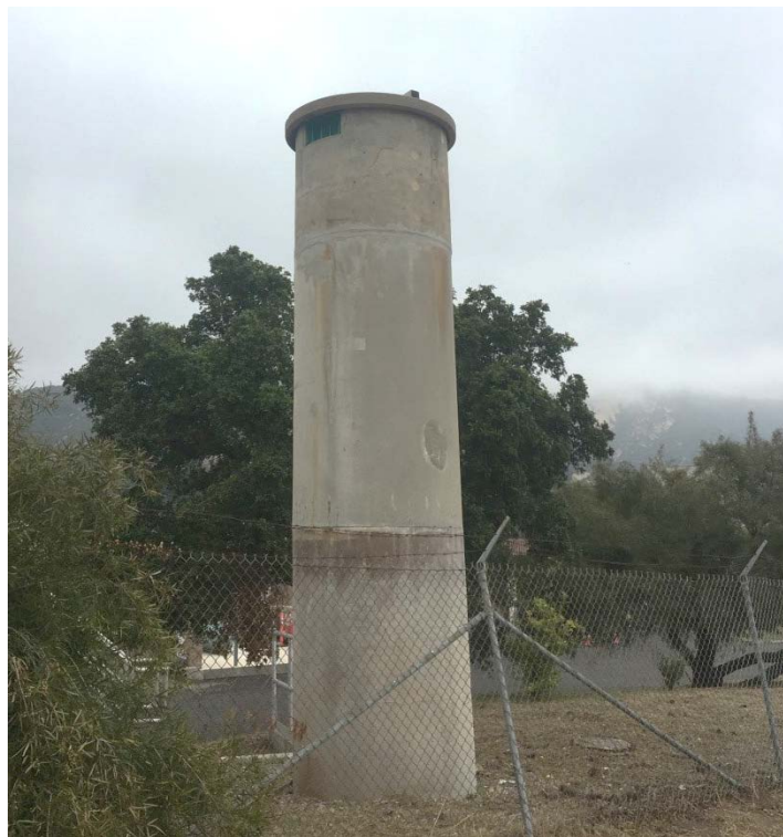
Top vault section replaced with vents and lid epoxy coated.
