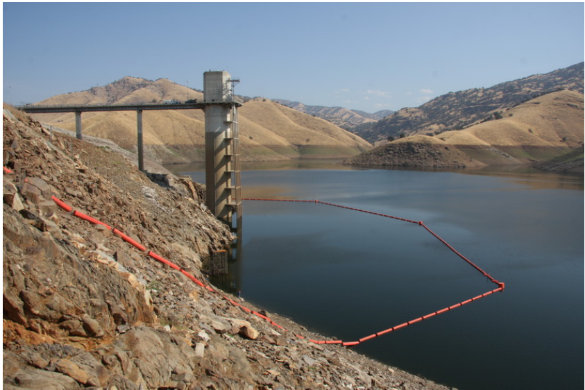
Figure 3. Intake Tower Protection with Debris Boom Lake Kaweah (Photo from TUFFBOOM)
