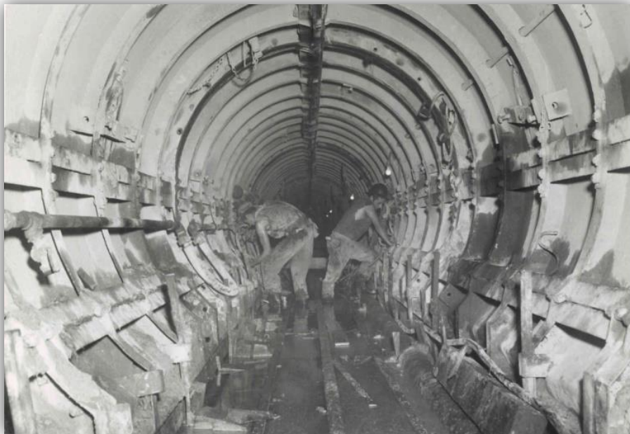
Tecolote Tunnel Construction
