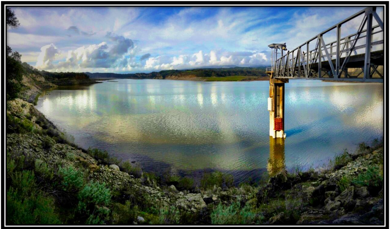
Cachuma Lake – North Portal Intake Tower Photo Credit: D. Flora
